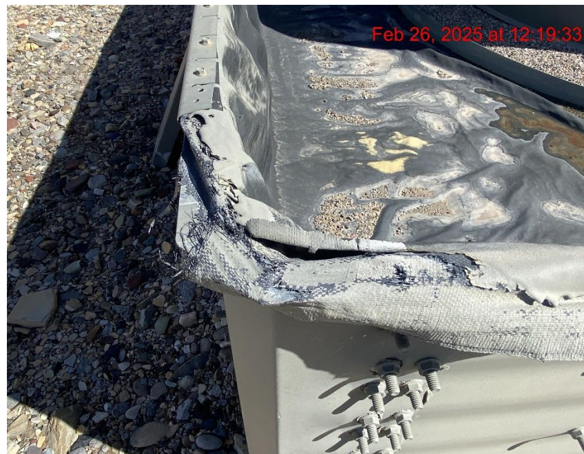
Berm Liner Separating From Containment – Photo #06881
