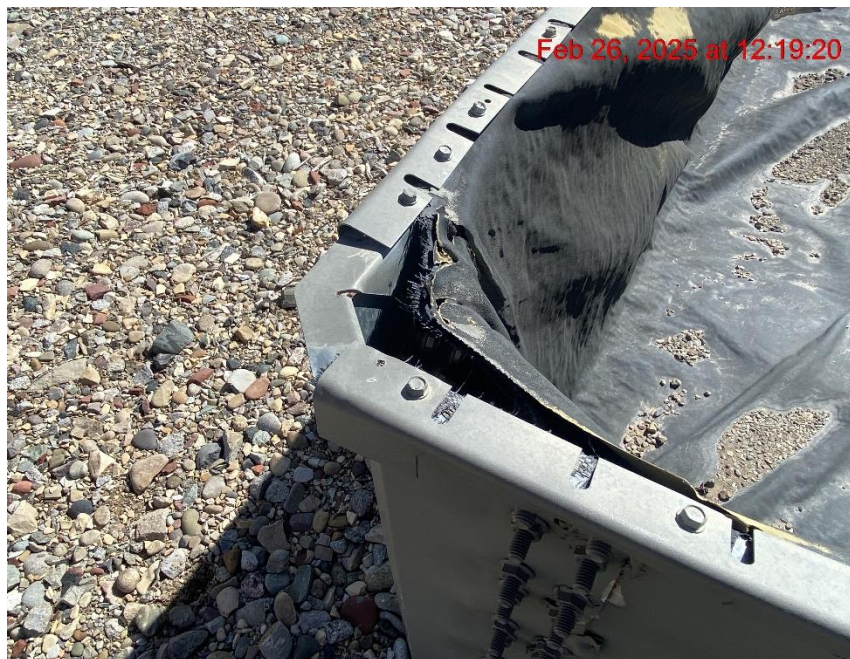
Berm Liner Separating From Containment – Photo #06880
