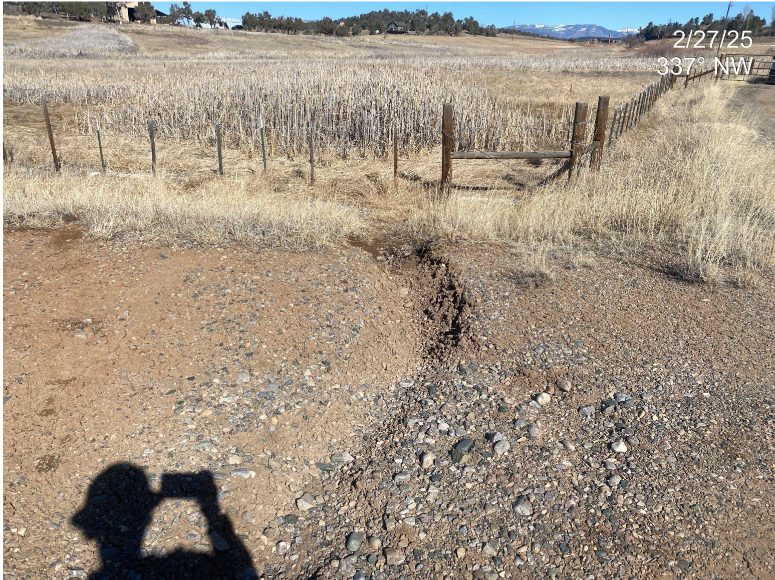
Photo 2. Erosion forming at the access point, BMPs needed in this area.
