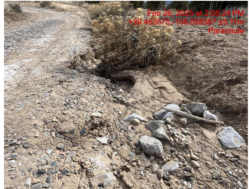
Photo # 5879 Erosion in ditch/road needs maintenance/insufficient BMP's
