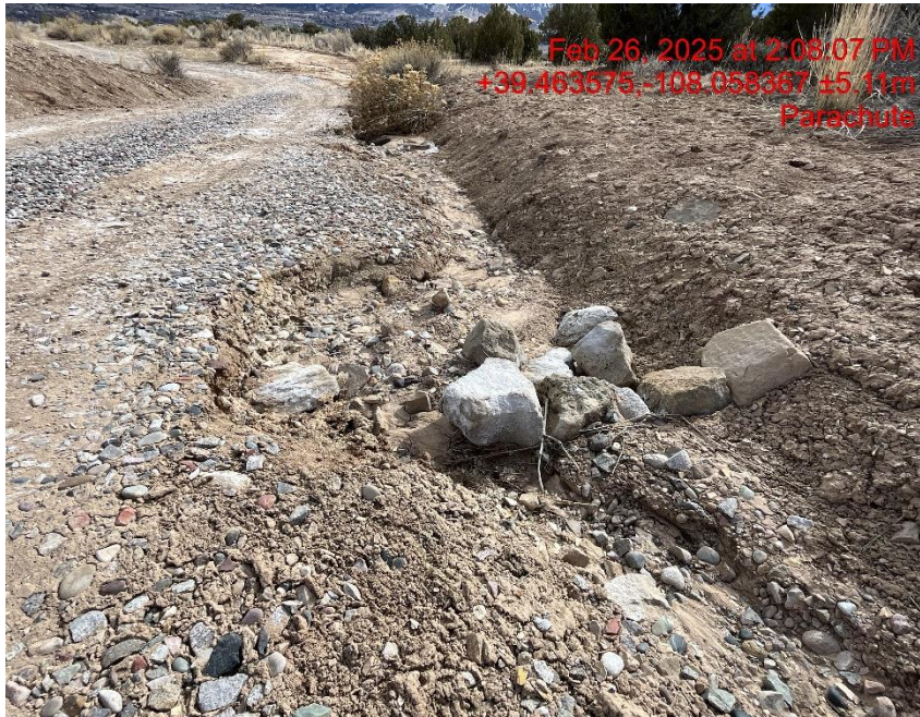
Photo # 5878 Erosion in ditch/road needs maintenance/insufficient BMP's
