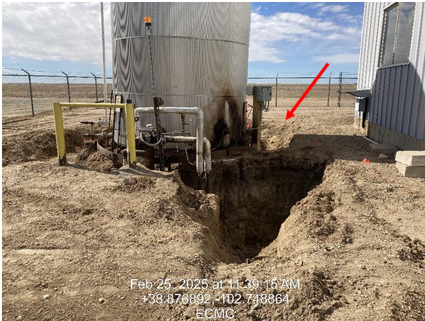
Photo 9 –Excavation area 2 at tank
