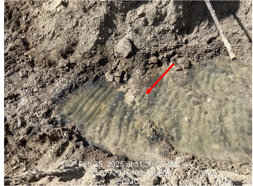
Photo 6 – Impacted soils in excavation, water was present at the time of inspection.
