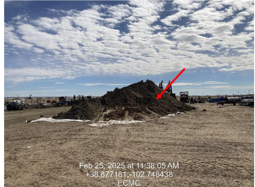
Photo 8 – Spoil pile on liner
