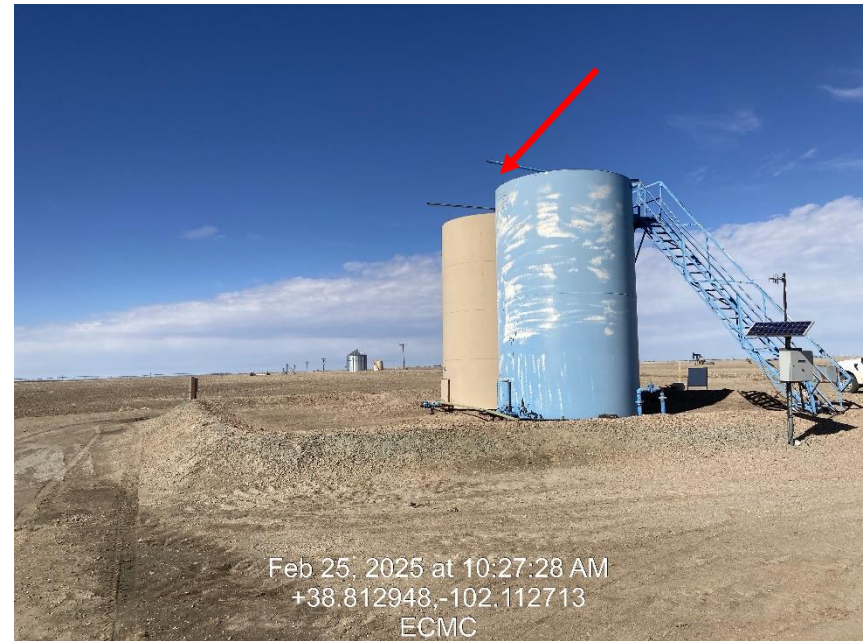
Photo 10 – Tank battery and equipment
