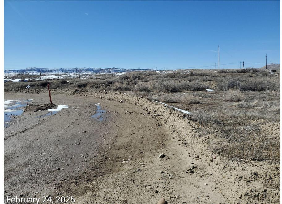
**Photo 2:** See comments under photo 1. Photo left also shows stabilization/tracking controls on the Location show sign of disrepair; rutting becoming evident.
