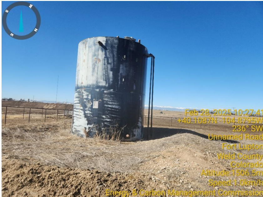
Photo 7 Tank battery no signage, berms need work.
