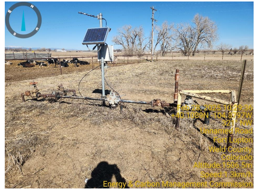
Photo 2 Gas Meter run not calibrated.
