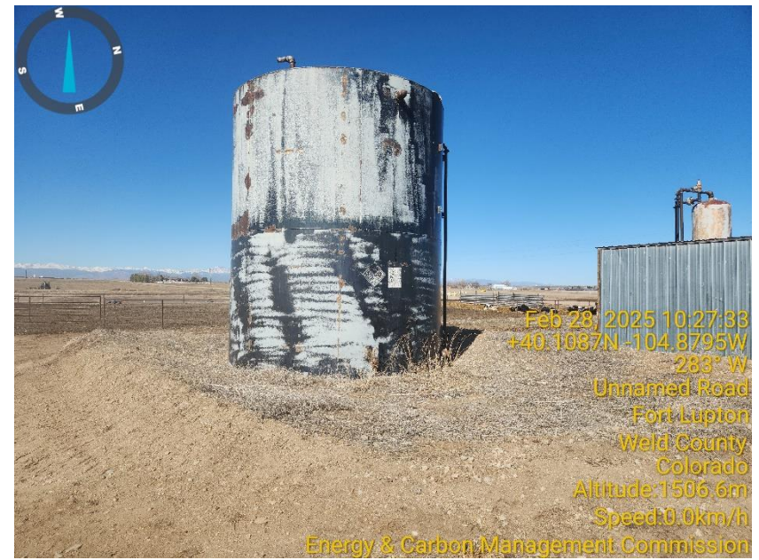
Photo 8 Tank battery no signage, berms need work.
