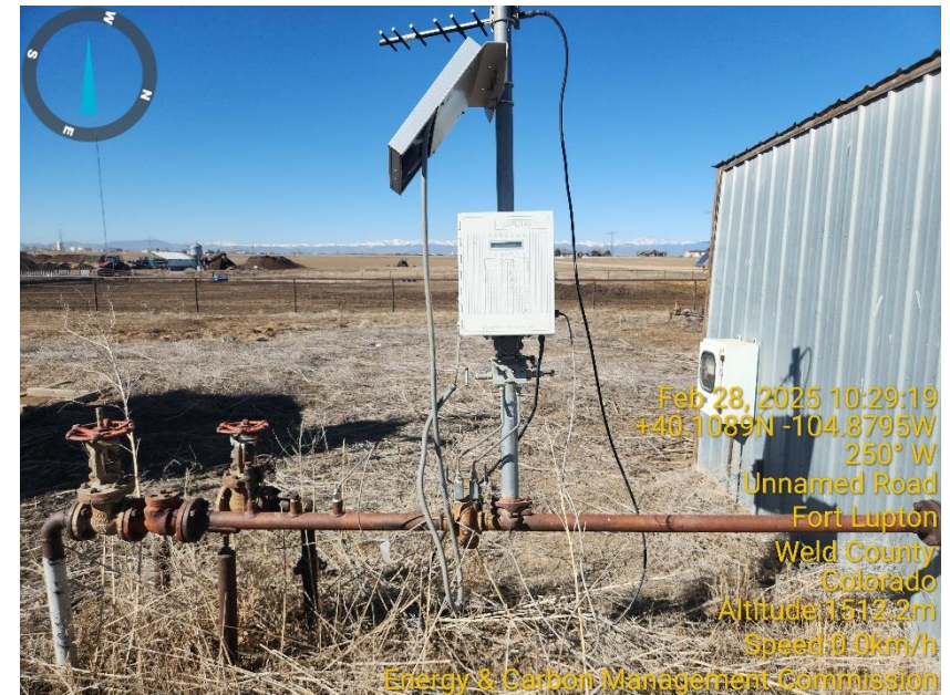
Photo 4 Dead vegetation around Gas Meter run not calibrated.
