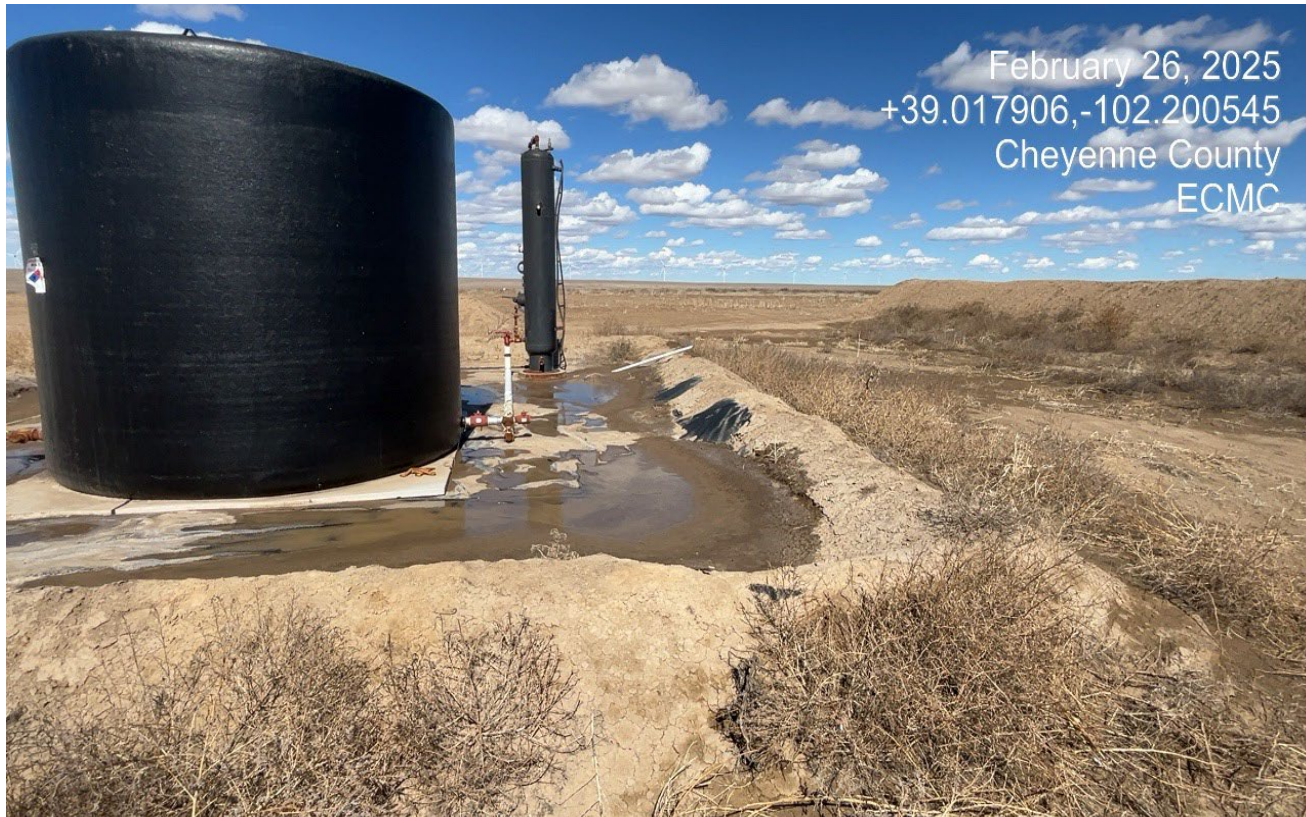
Photo 2. The berm is worn down in this area. This berm is not designed to resist degradation from erosion and there are weeds growing along the berm.
