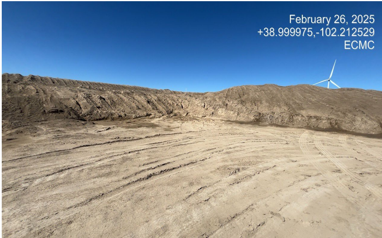
Photo 4. Facing toward the northeast side of the location. There is erosion along the topsoil pile which is mixing soil into the pad surface and subsoils. The topsoil is not stabilized or protected.
