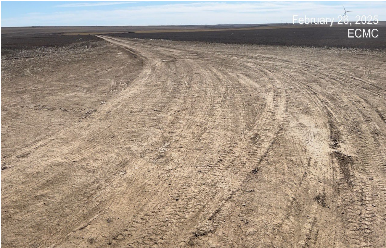
Photo 1. Facing south along the access road. The access road needs to be reduced in size by reclaiming and decompacting soils.
