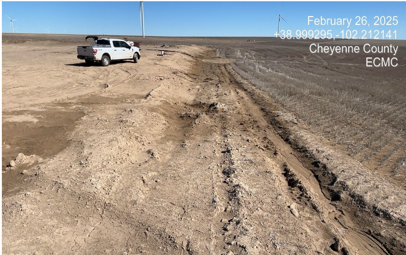
Photo 10. Facing east along the south side of the location. There are insufficient BMP's on the down hill side to stormwater control. The perimeter ditch has filled in with sediment.
