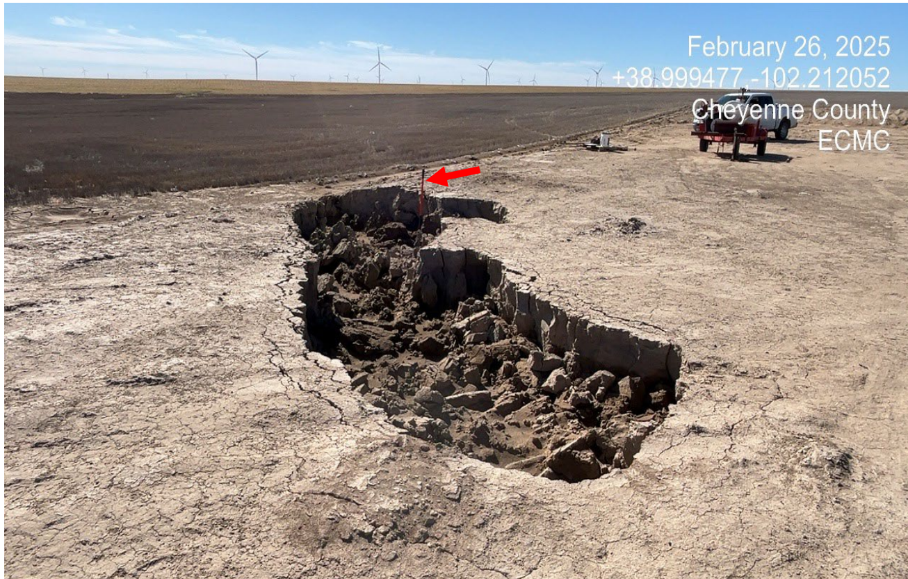
Photo 7. There is significant gully erosion along the fill slope which has washed sediment out into the adjacent crop field. Red arrow points to 4.5 ft. shovel. Previous CA was not completed.
