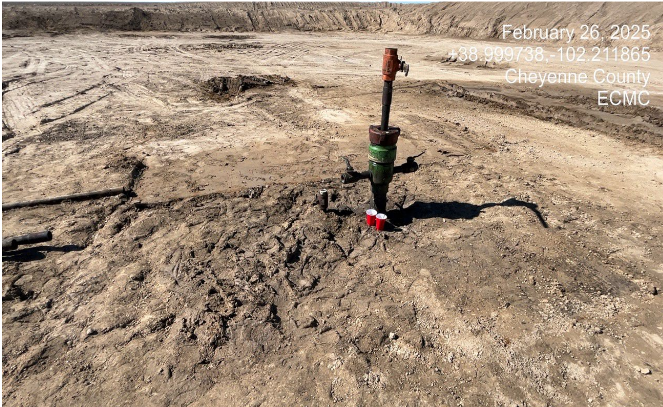
Photo 6. Facing toward the wellhead. There are stained soils around the wellhead.
