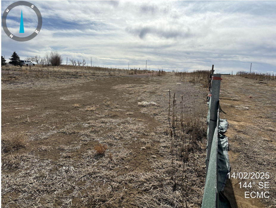
Photo 1. Looking south towards access road. It appears that gravel was removed from the well location and that reclamation work was conducted. The remaining access road is being used as a driveway.
