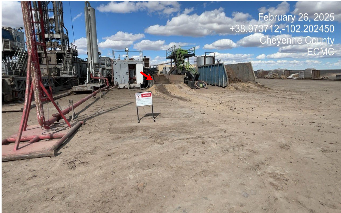
Photo 8. Facing north toward the drill rig and cutting/ mud management area. A loader was moving the drill mud/cuttings from the container at red arrow and tracking the E&P waste over to the containers shown in the next photo.
