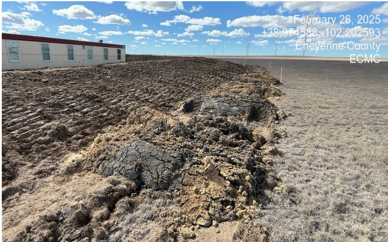
Photo 16. Facing toward the northwest side of the location. There is more drill cuttings and mud that was dumped along the back side of the topsoil pile. E&P waste is not being properly handled and disposed and has caused further contamination on the surface.
