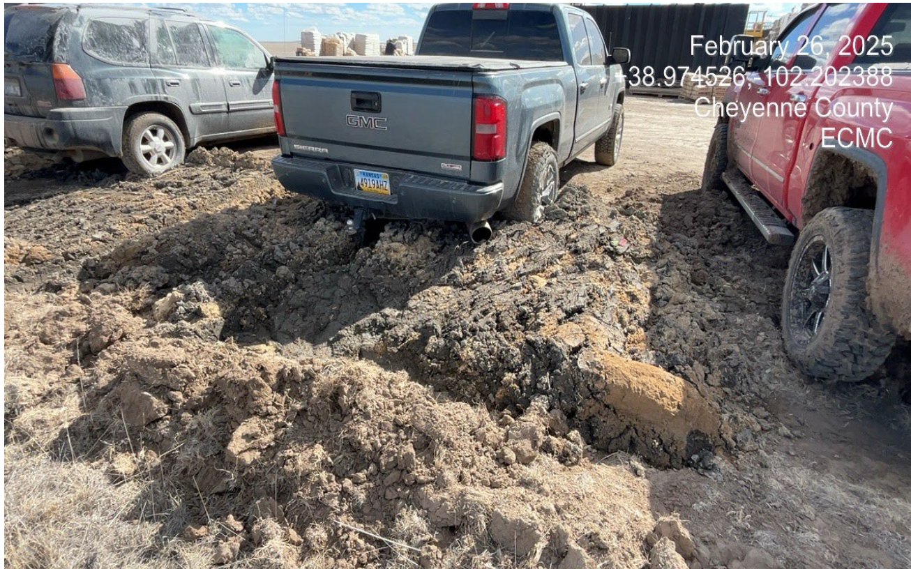
Photo 15. Vehicles are parking and tracking the drill cuttings and mud that was dumped in this area. E&P waste is not being properly handled and disposed and has caused further contamination on the surface.
