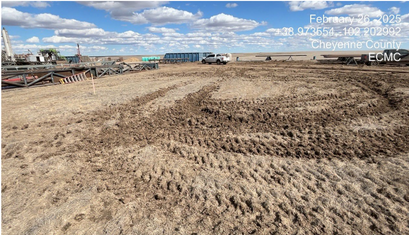
Photo 6. Vehicles and equipment were driving off the road and location causing unnecessary disturbance.
