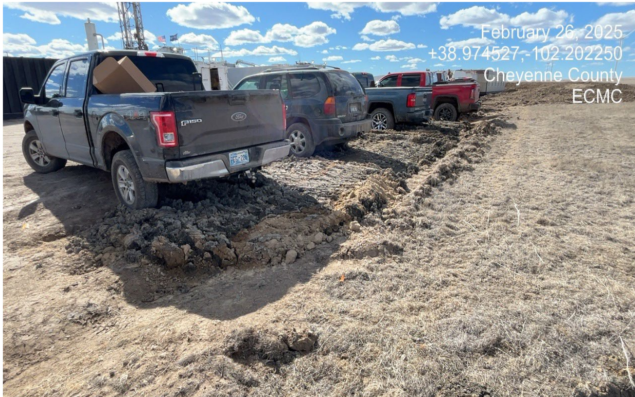
Photo 14. North side of the location facing southwest. The perimeter stormwater ditch has been filled in. The material that was dumped in this area is greyish with sawdust resembling drill cuttings and mud.
