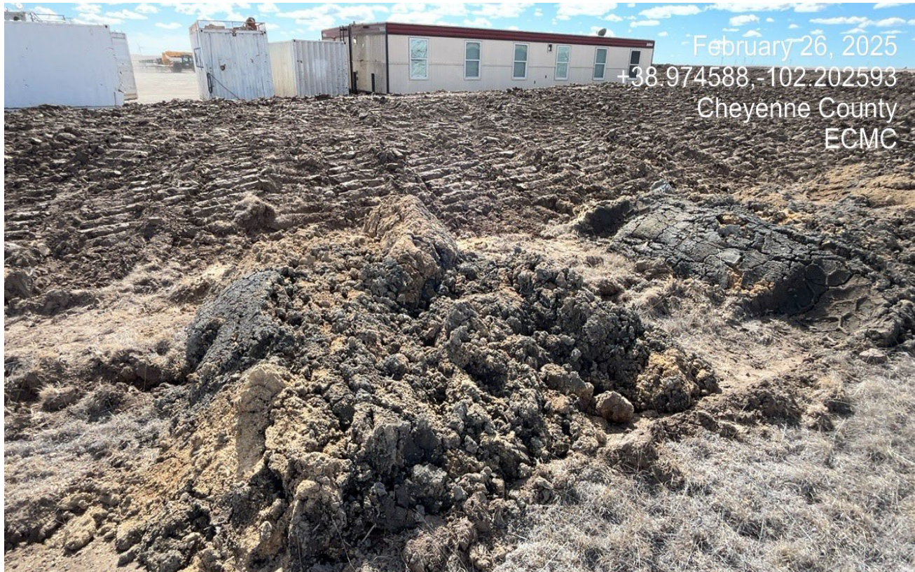
Photo 17. View of drill cuttings and mud that was dumped along the back side of the topsoil pile. E&P waste is not being properly handled and disposed and has caused further contamination on the surface.
