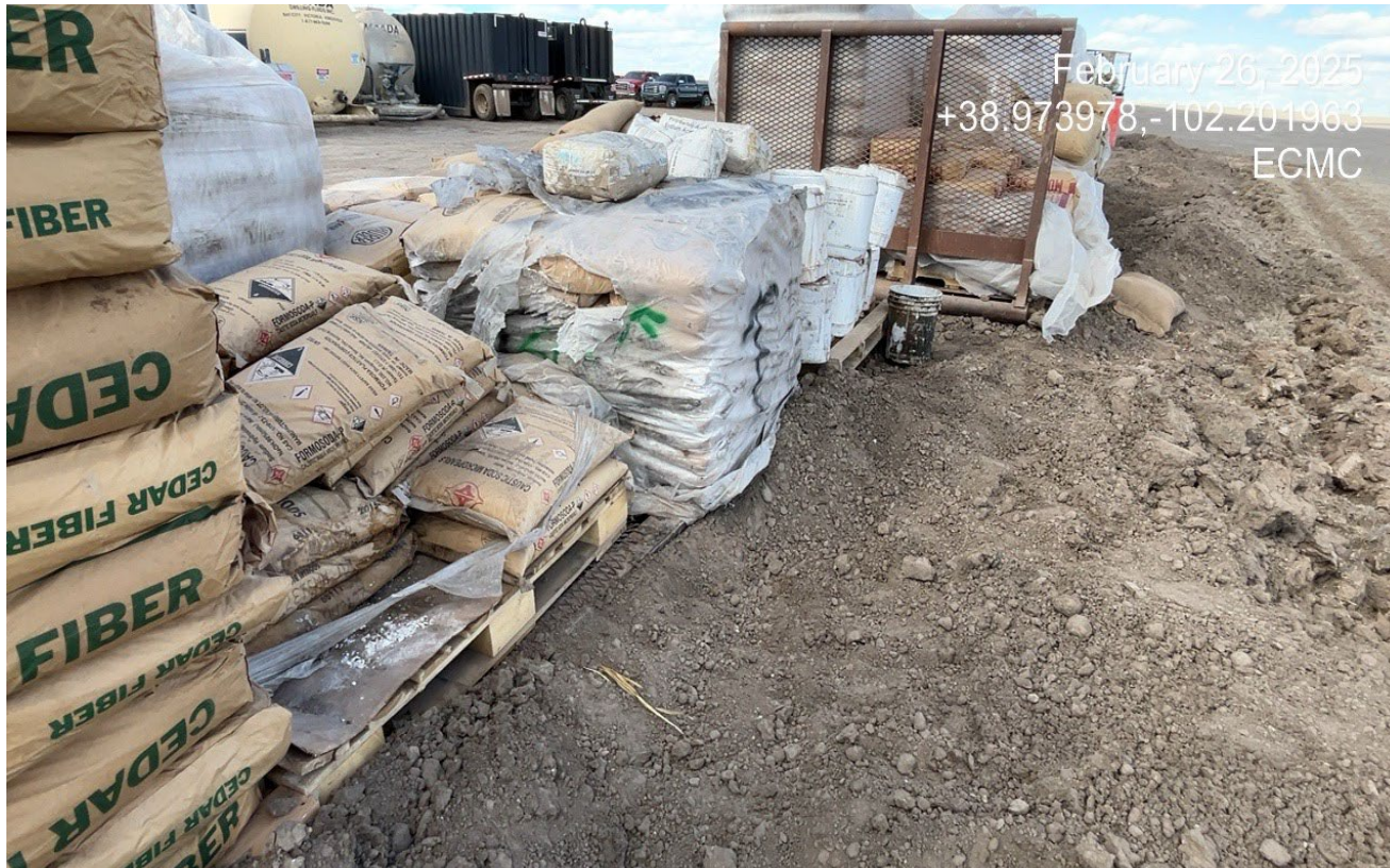
Photo 12. The bags of chemical products are not stored with containment and some of the contents have spilled onto the ground.
