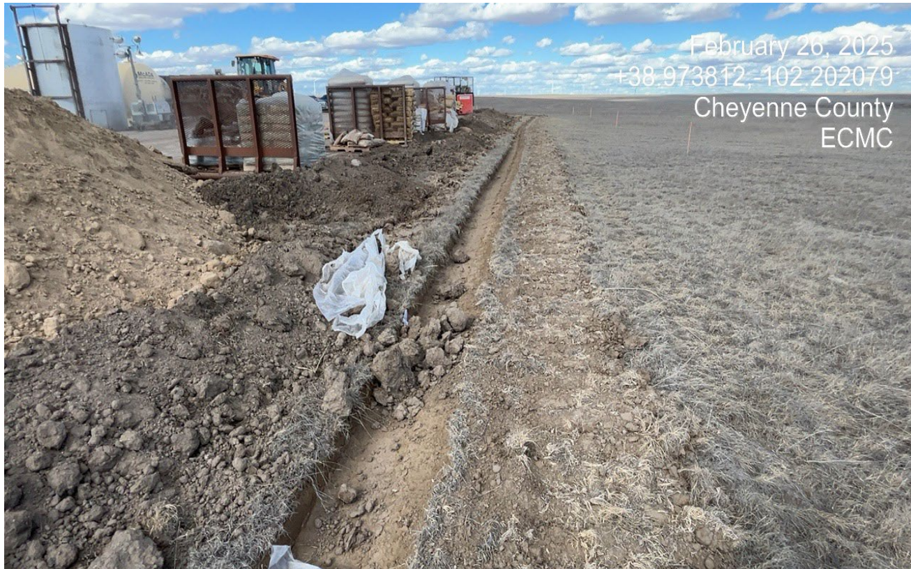
Photo 11. East side of the location facing north. There is trash debris not contained and dirt clouds have fallen into the stormwater ditch.
