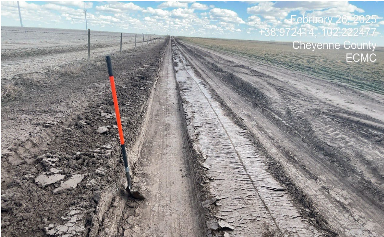
Photo 1. Facing east along the access road. The road has become rutted and damaged due to driving in wet conditions without adequate BMP's
