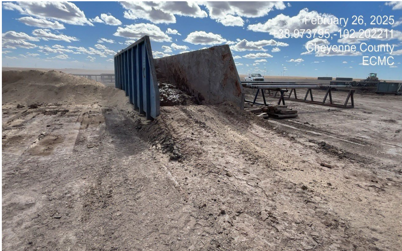
Photo 10. The drill cuttings/mud is being mixed with sawdust on the left and dumped into this open end container. The mud is being tracked along this area and onto the surface. E&P Waste management is not being performed in a protective manner.
