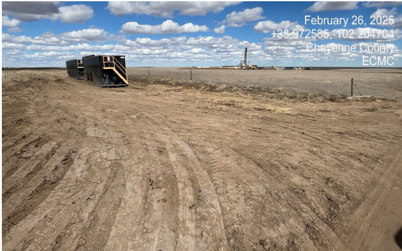
Photo 4. There has been unpermitted disturbance which has occurred where vehicles and equipment were parking off the location. This area will need to be reclaimed.
