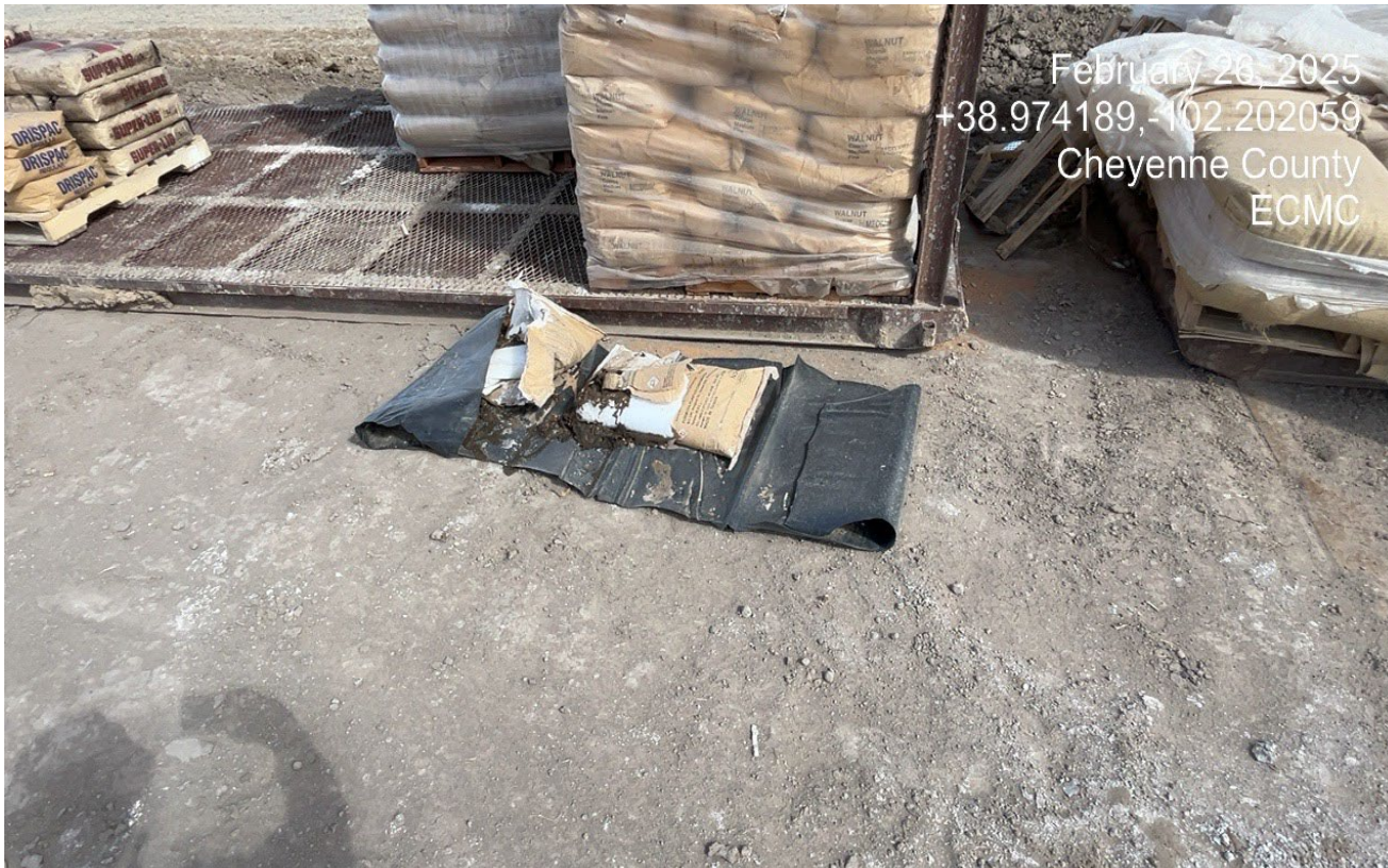
Photo 13. The bags of chemical products are not stored with containment and some of the contents have spilled onto the ground.
