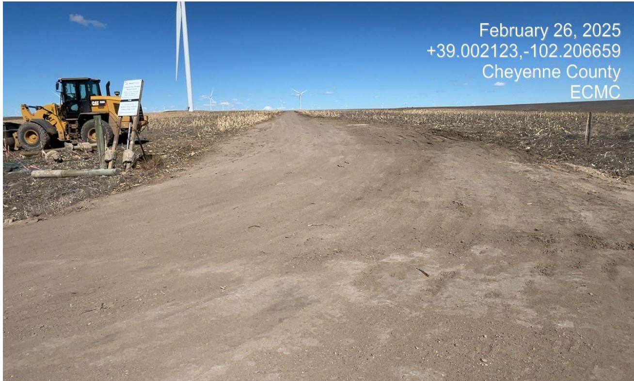
Photo 1. Facing north toward the access road.
