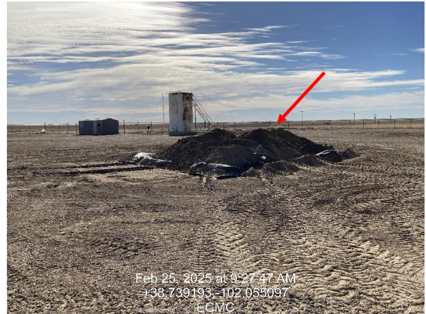
Photo 6 – Contaminated soils stored on liner
