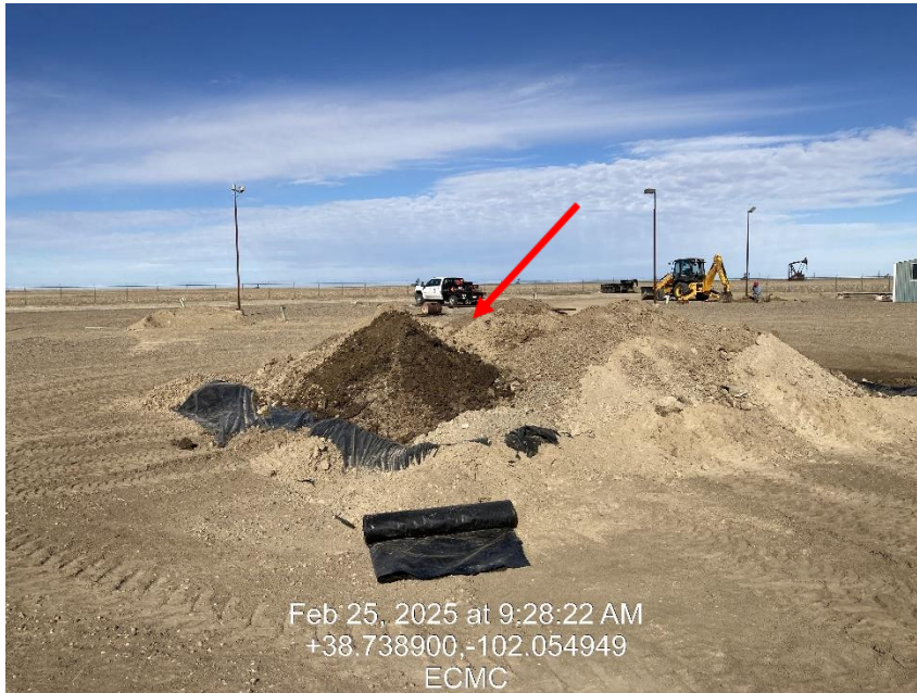
Photo 7 –Contaminated soils stored on liner
