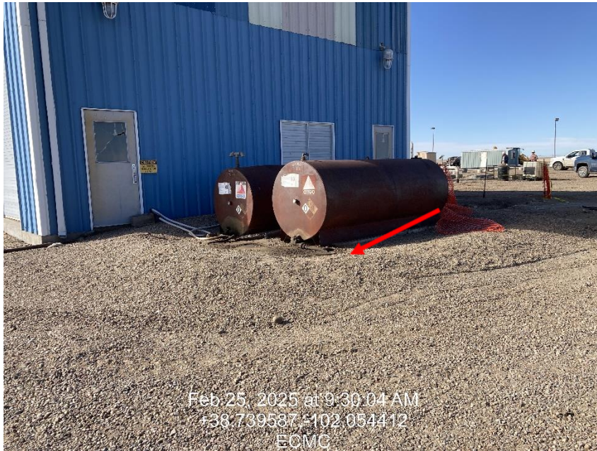
Photo 11 – Tanks with stained soils no secondary containment
