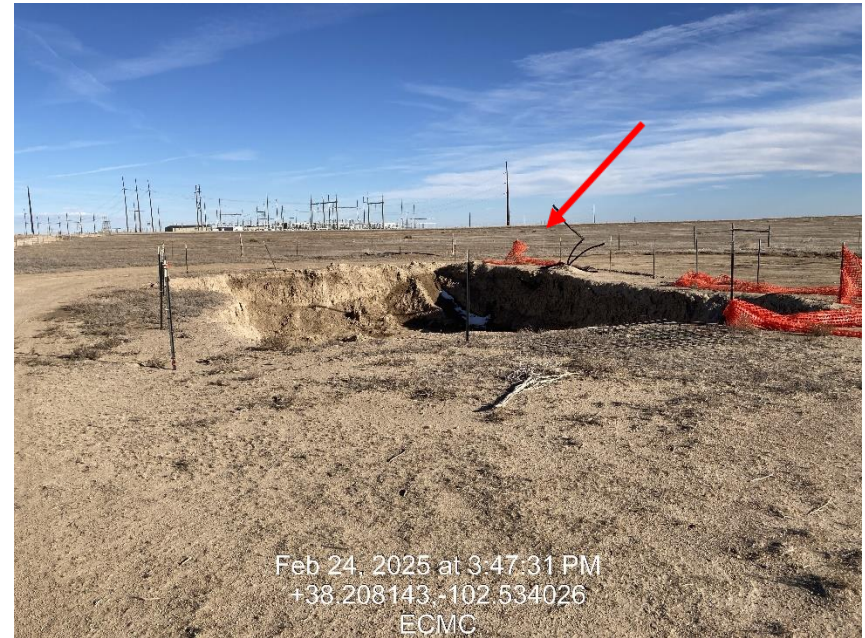
Photo 6 – Remediation area at tank battery, temporary fence is not adequate
