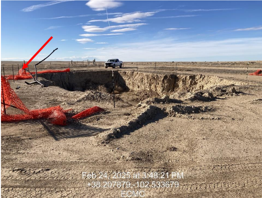
Photo 7 – Remediation area at tank battery, temporary fence is not adequate
