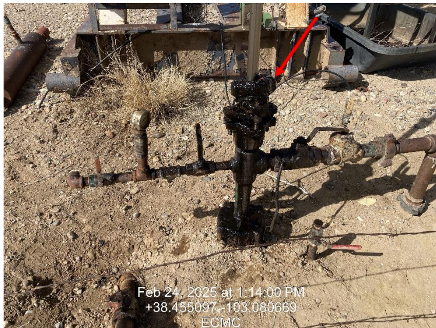
Photo 3 – Wellhead covered in oily sludge
