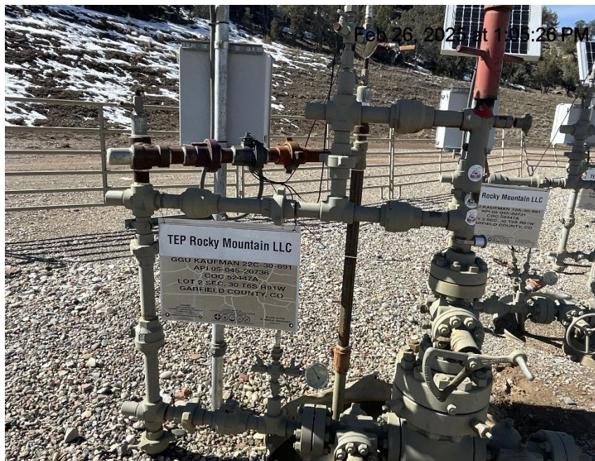
Photo # 9307 Wellhead signs missing required information
