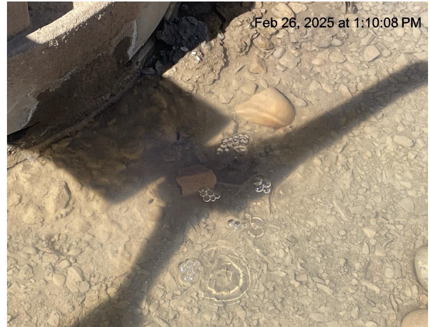
Photo # 9302 Mechanical Condition - Possible wellhead leak /gas bubbling up through water in cellar (GGU Kaufman 22C-30-691)
