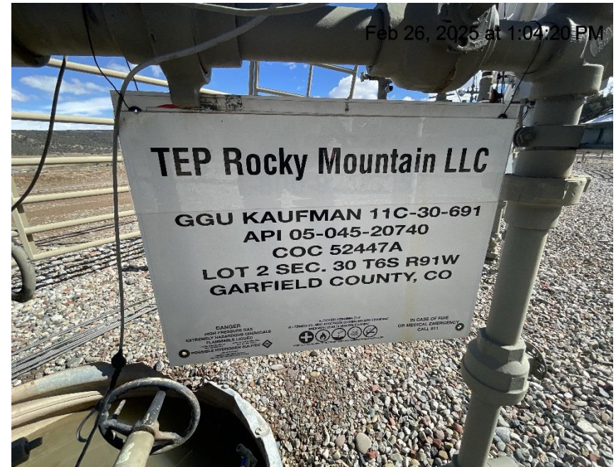
Photo # 9304 Wellhead sign missing required information
