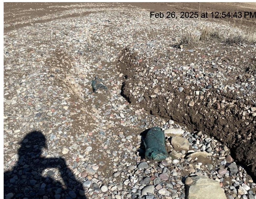
Photo # 9316 Ditch & check dams need maintenance
