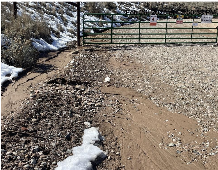
Photo # 9309 Ditch needs maintenance
