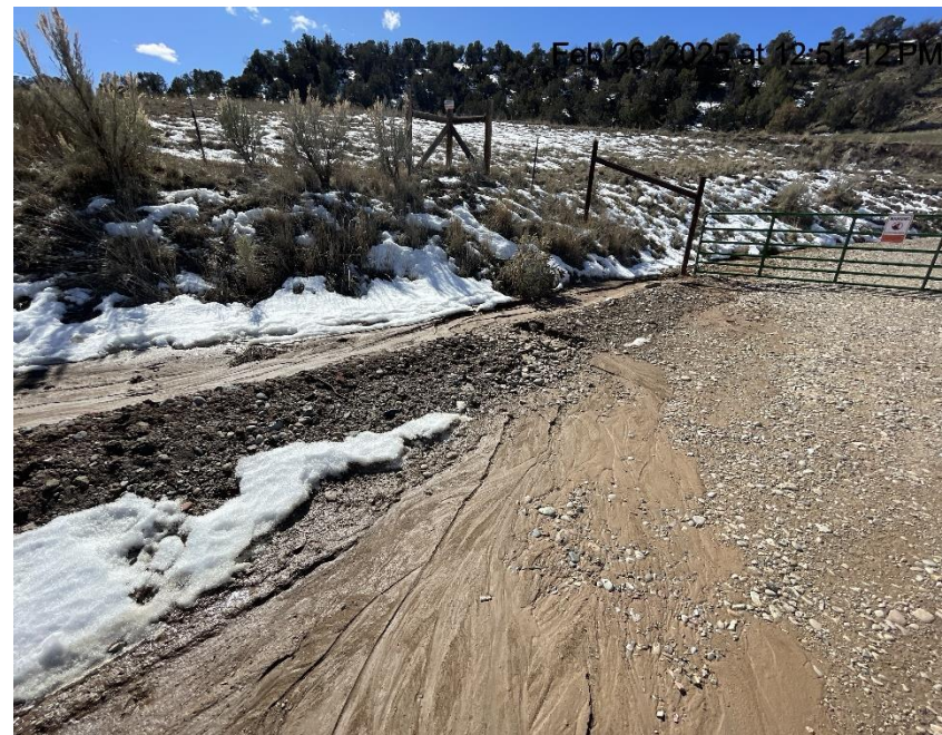
Photo # 9310 Ditch needs maintenance
