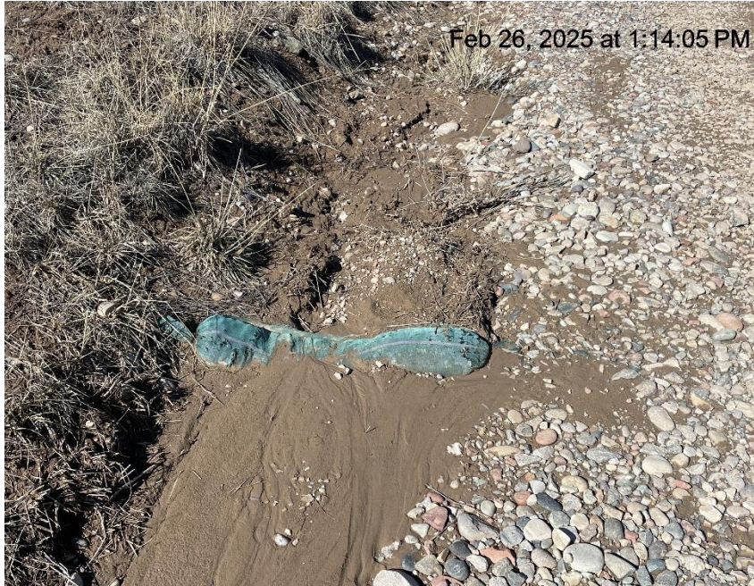
Photo # 9319 Ditch & check dams need maintenance
