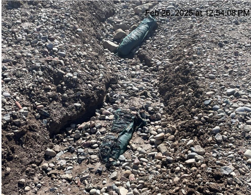
Photo # 9317 Ditch & check dams need maintenance
