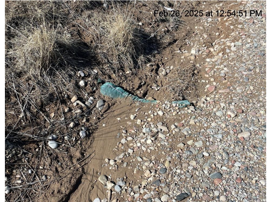
Photo # 9318 Ditch & check dams need maintenance
