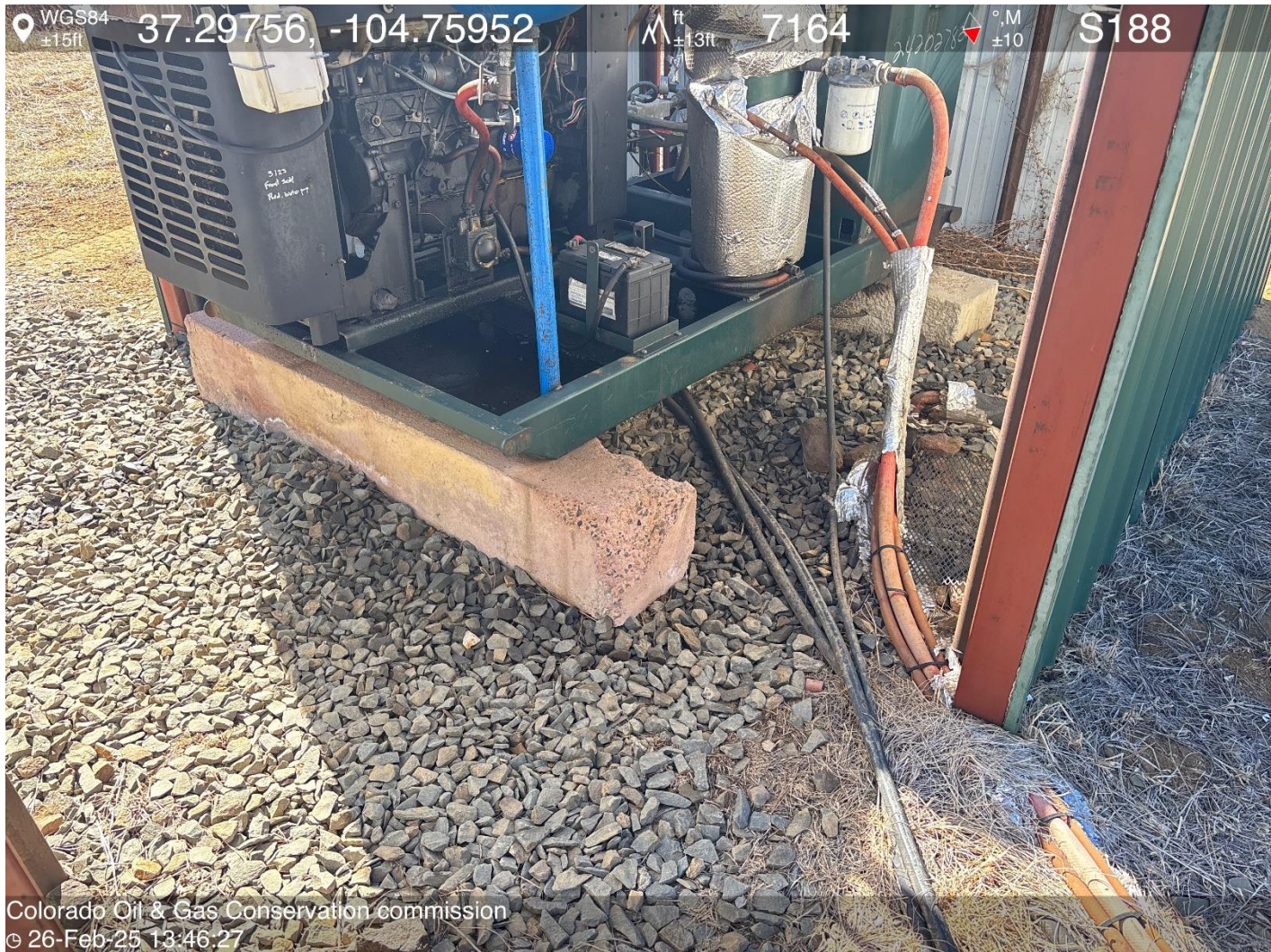
PHOTO 5: THERE IS AN AREA OF IMPACTED SOIL NEAR PRIME MOVER ENGINE SKID. Conduct maintenance on equipment (REPAIR LEAKS), cleanup stained material and review self inspection processes. COMPLY WITH RULE 1002,(2).D CA DATE 3-5-2025.
