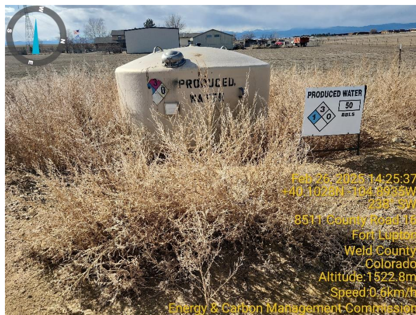
Photo 6 Produced water tank.
