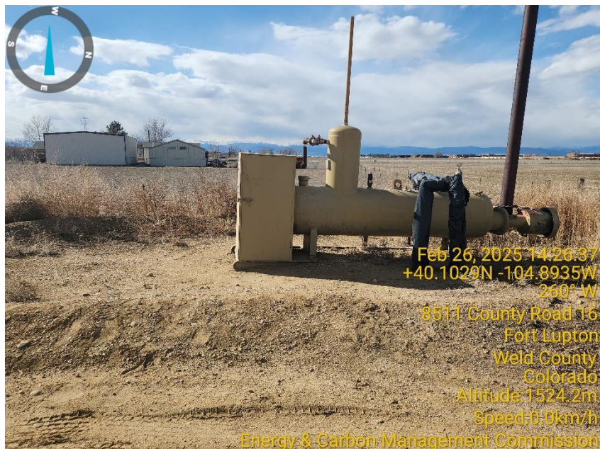
Photo 7 Horizontal heated Separator.
