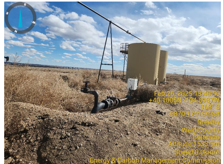
Photo 10 Gas Meter Run.
