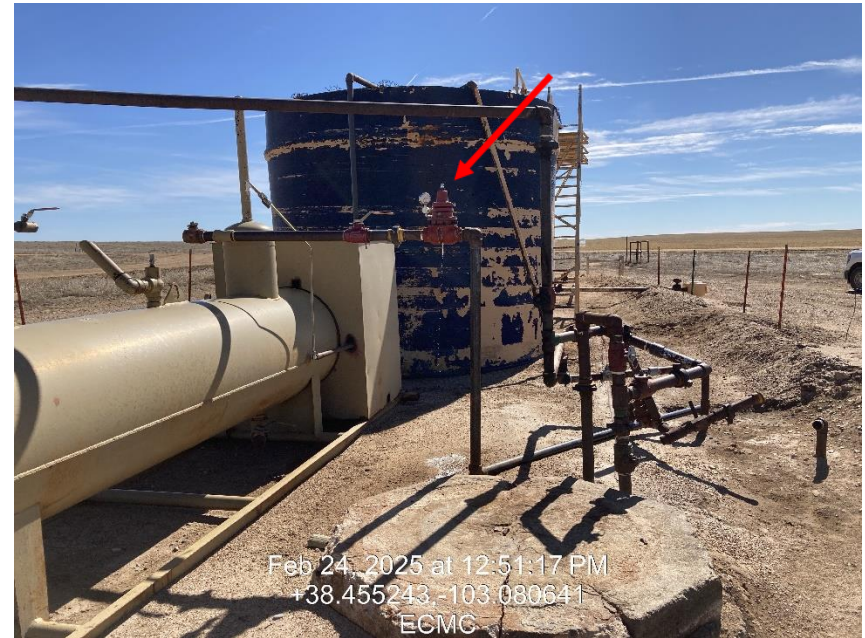
Photo 6 – Leaking valve
