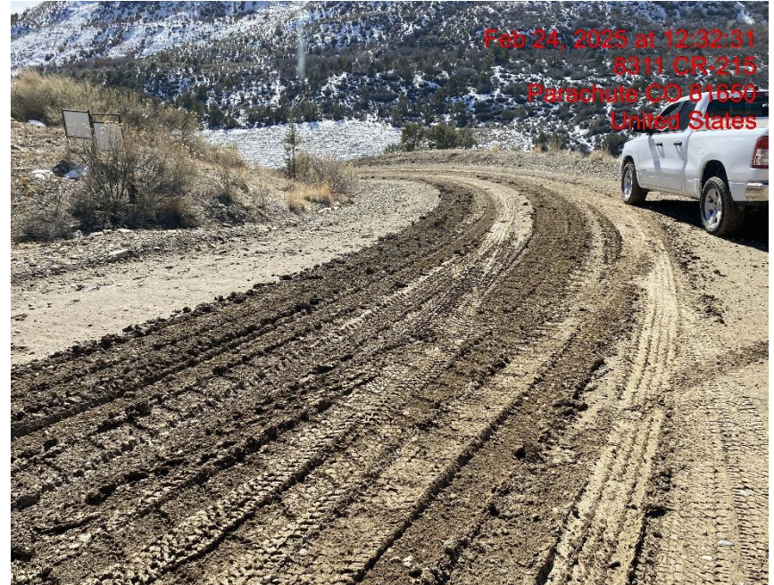
Insufficient Tracking BMPs – Photo #06835
