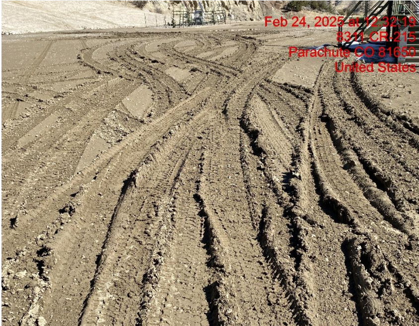
Lack of Stabilization – Photo #06834
