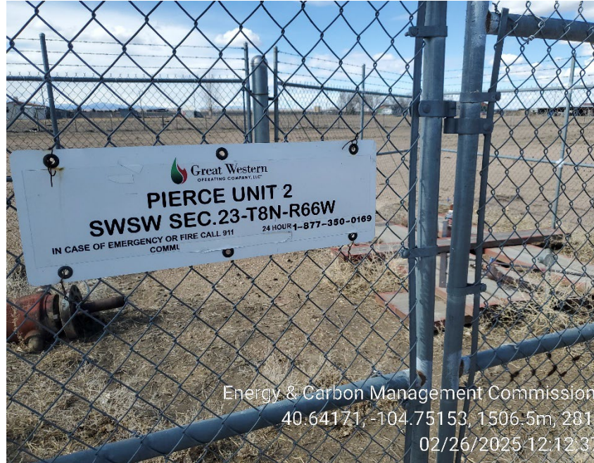
Wellhead and sign
