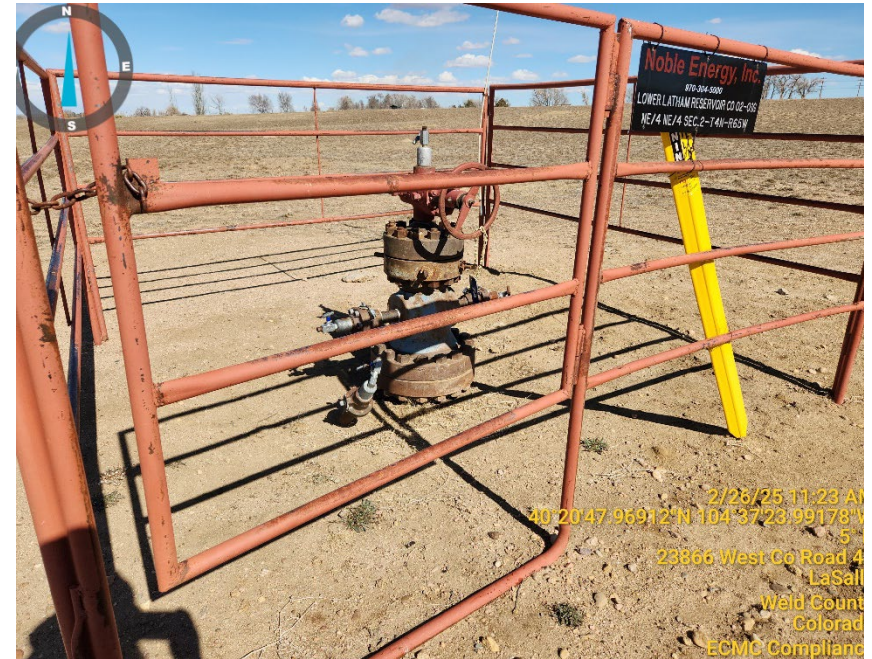
Photo 2: TA Wellhead
