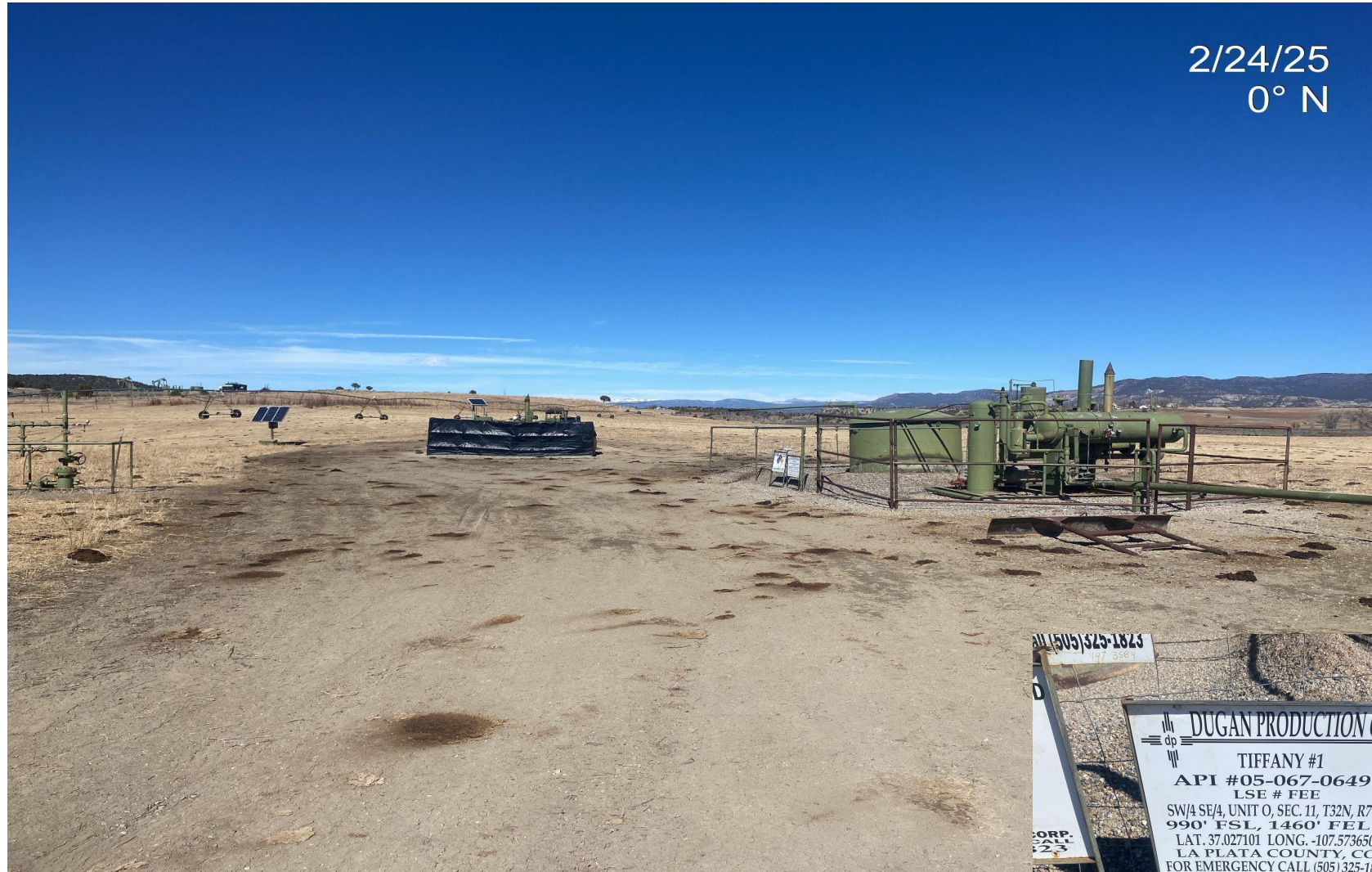
Photo 1. View of the well pad taken from the access point facing center. Note: no local emergency services number displayed on location sign.
