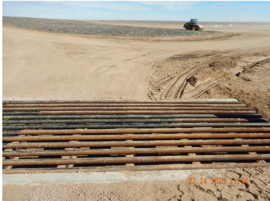
Photo 2. Photo taken west of the entrance to location, facing Northeast. Photo illustrates the Operator has installed a vehicle tracking control (VTC) device BMP. Operator plans to install an addition VTC near the Operator sign shown in Photo 1.
