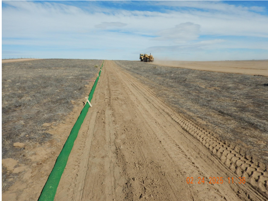
Photo 4. Photo taken from the western portion of location, facing North. Photo illustrates a perimeter stormwater BMP (ditch and berm with filtrex wattles) have been installed along the entire perimeter of location.
