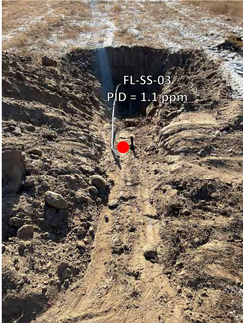
Looking southwest at bellhole/change in direction
