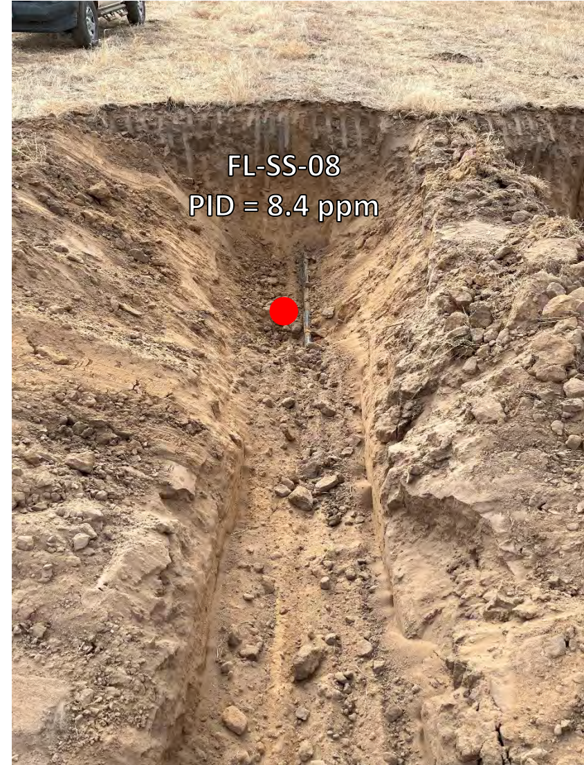
Looking southwest at bellhole/change in direction
