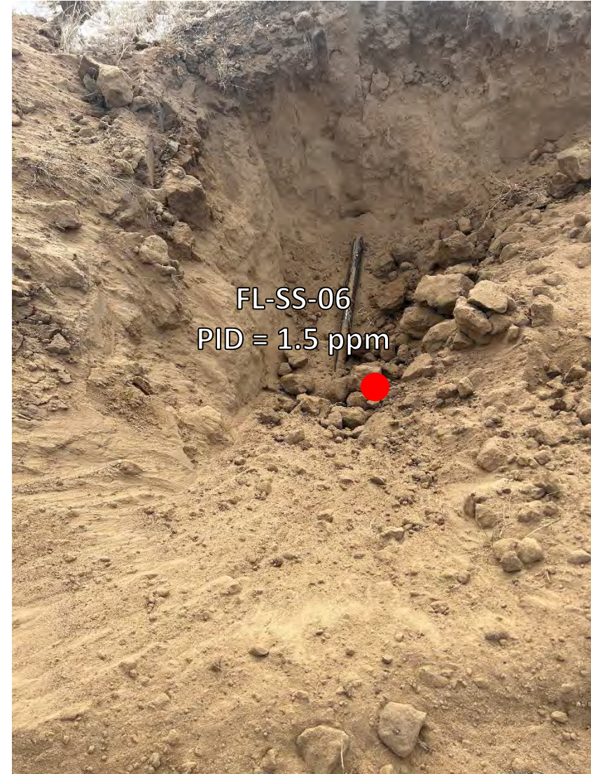
Looking south at bellhole/change of direction
