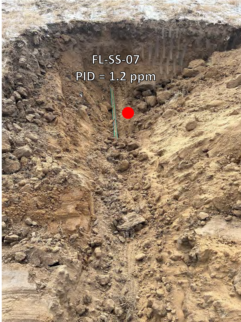
Looking south at bellhole/cut point for removal
