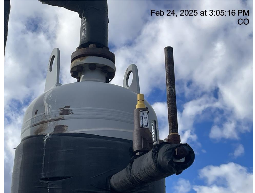
Photo # 8635 PRV vent line does not comply with CECMC pressure safety device rules
