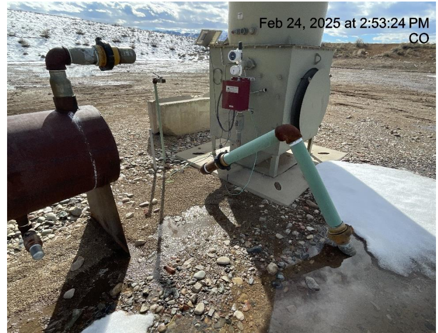
Photo # 8637 ECD completely disconnected & not in use /unused equipment
