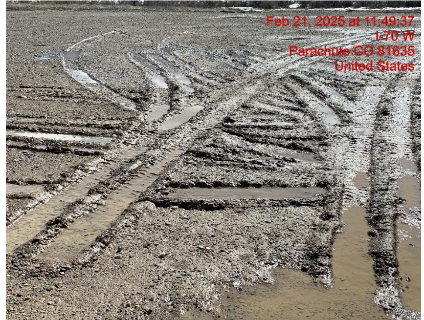
Lack of Stabilization – Photo #06810
