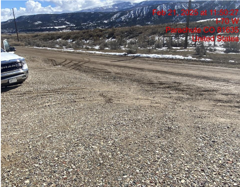
Insufficient Tracking BMPs – Photo #06812
