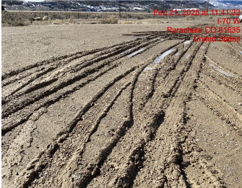
Lack of Stabilization – Photo #06799
