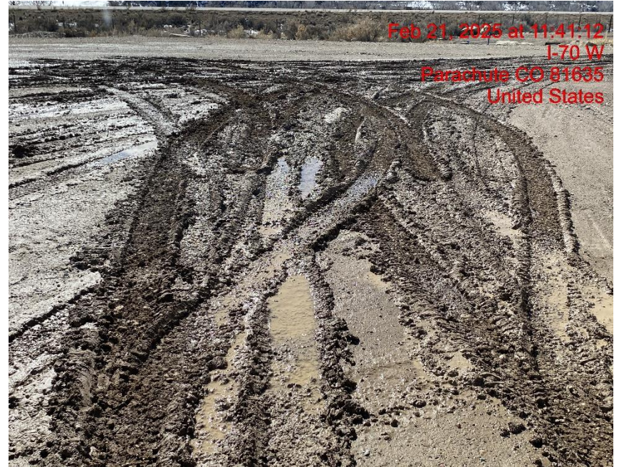
Lack of Stabilization – Photo #06798
