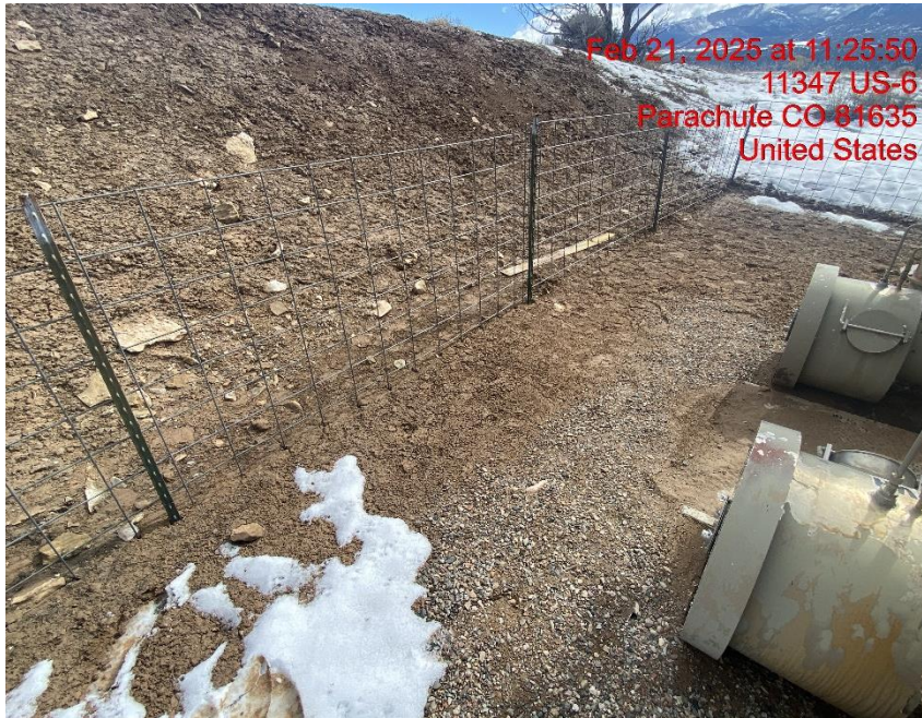
Insufficient Erosion Control – Photo #06786
