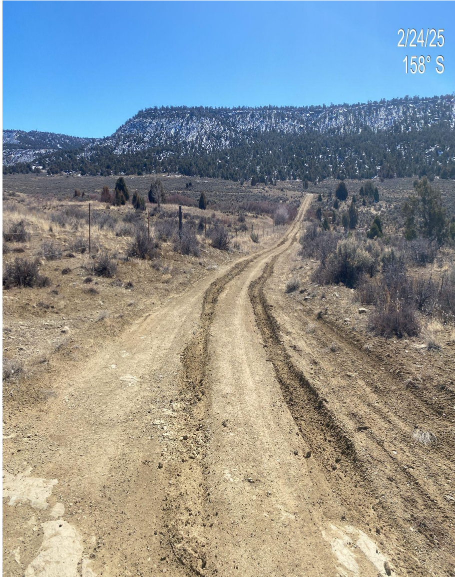
Photo 2. Rutting observed at access road and along perimeter of pad.
