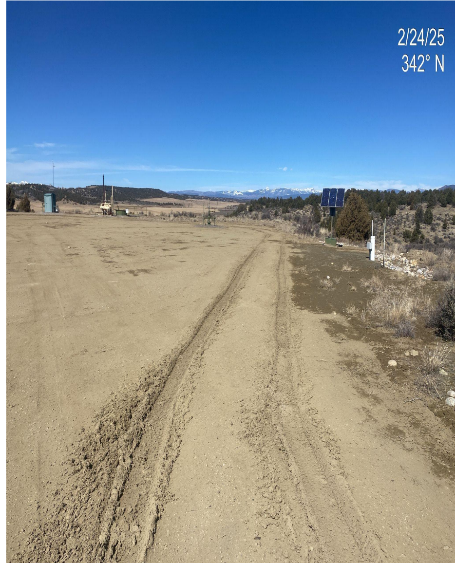
Photo 2. Rutting observed at access road and along perimeter of pad.
