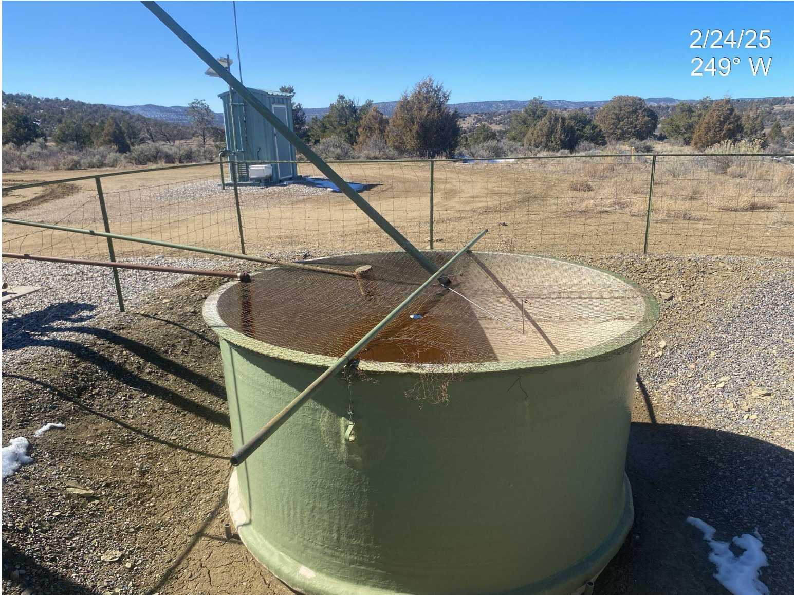
Photo 3. Wildlife netting at produced water tank has ripped and is no longer functioning.
