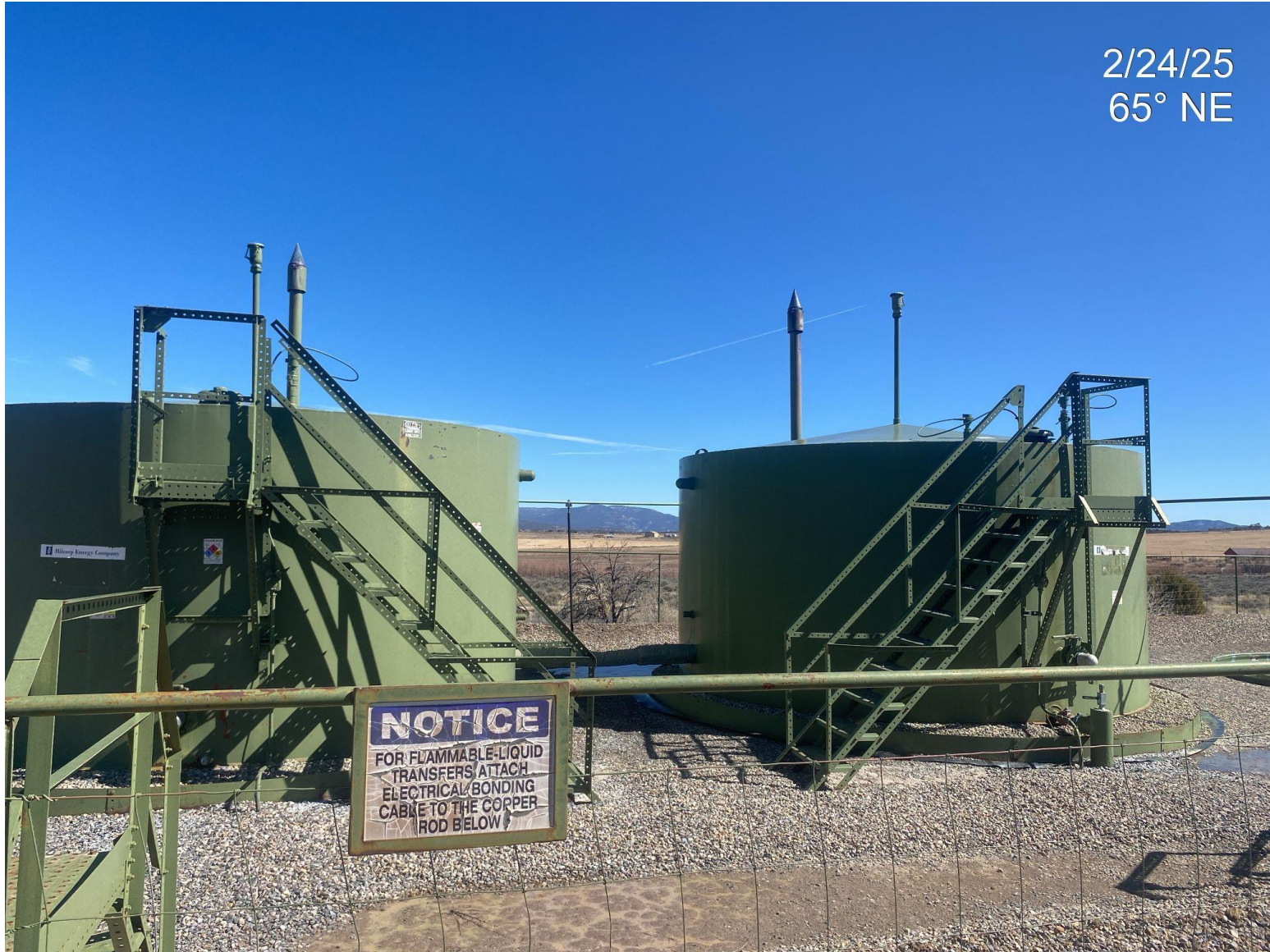
Photo 2. Capacity not displayed at produced water tank labels.
