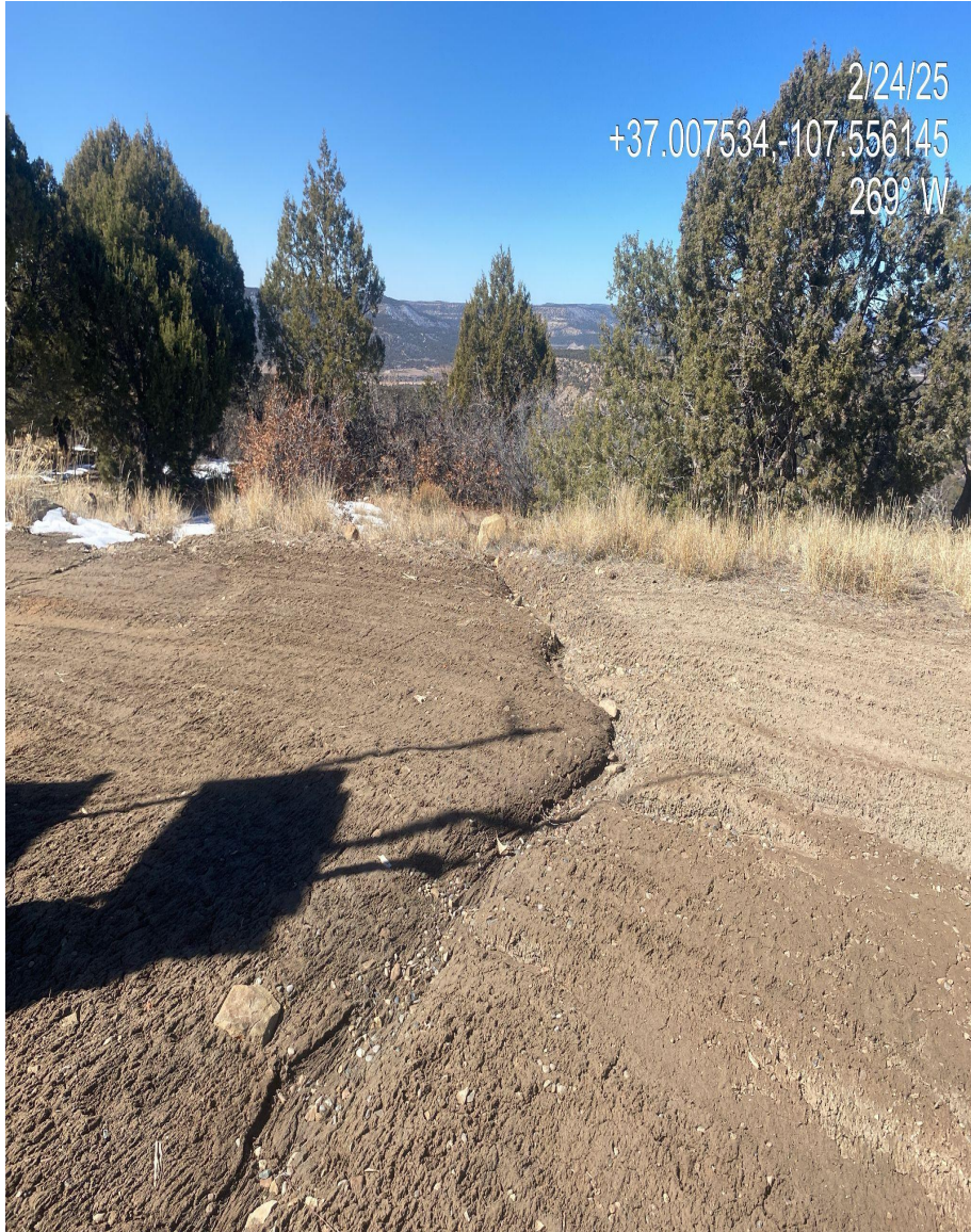
Photo 4. Erosion forming on the western edge of the pad.
