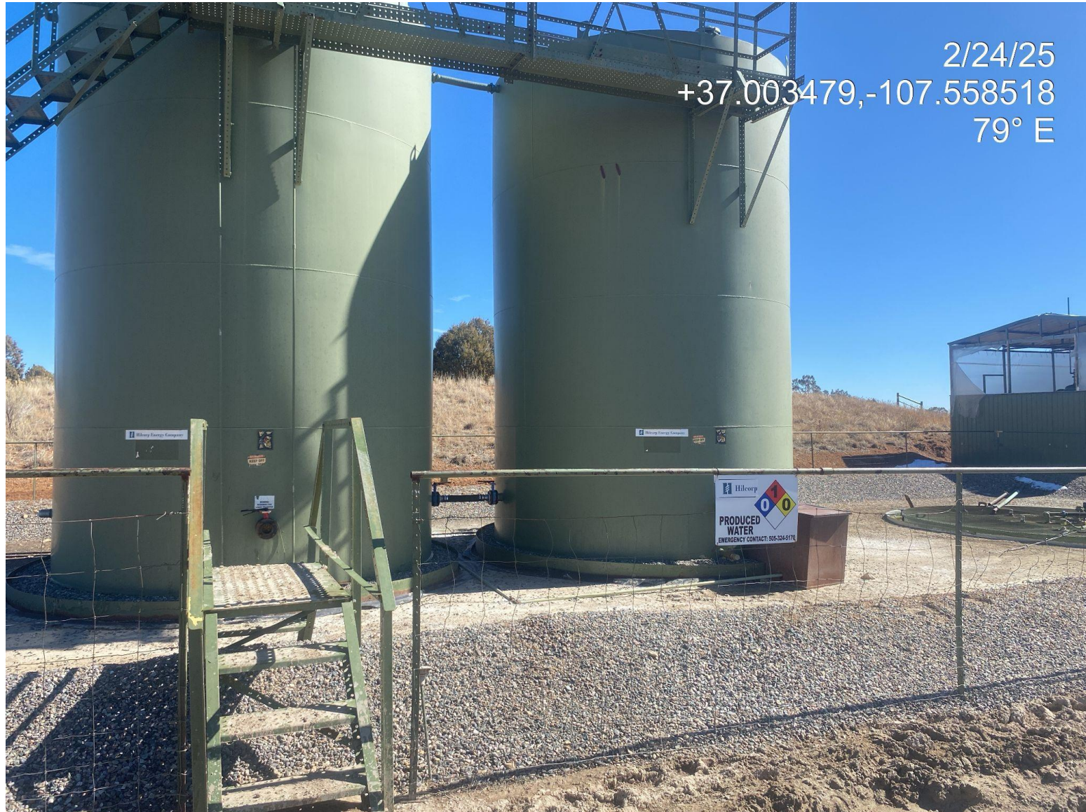
Photo 3. Produced water tanks labels are not displaying tank capacity.
