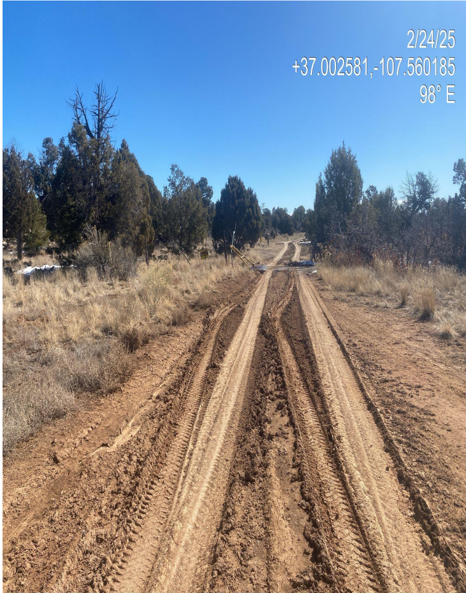
Photo 2. Rutting occurring on active pad, grading/stabilization required to minimize degradation to the active pad.
