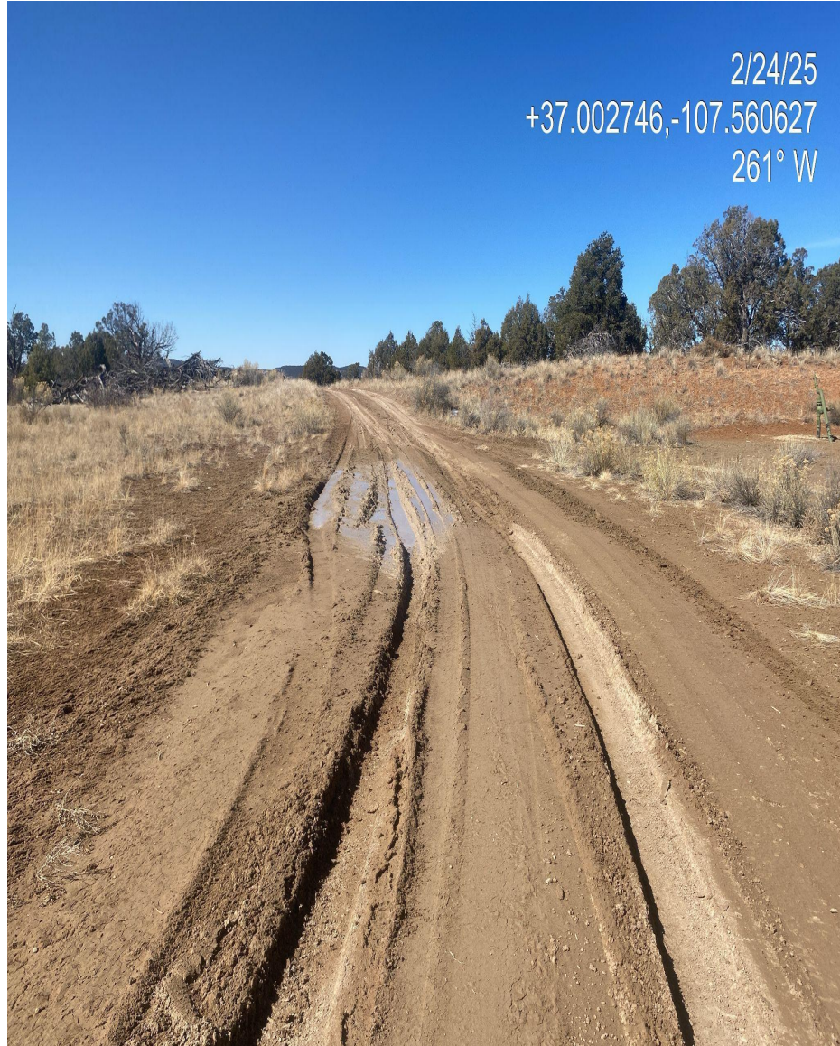
Photo 2. Rutting occurring on active pad, grading/stabilization required to minimize degradation to the active pad.
