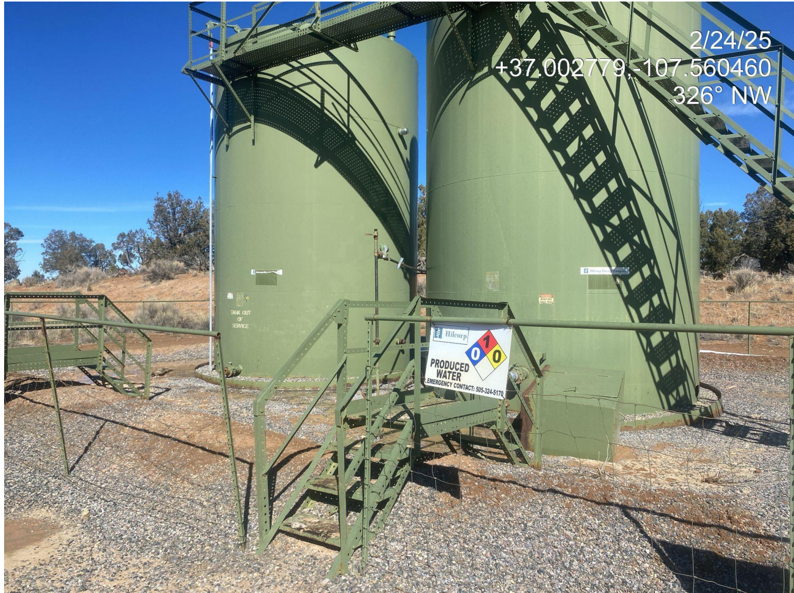
Photo 4. Produced water tanks labels are not displaying tank capacity.
