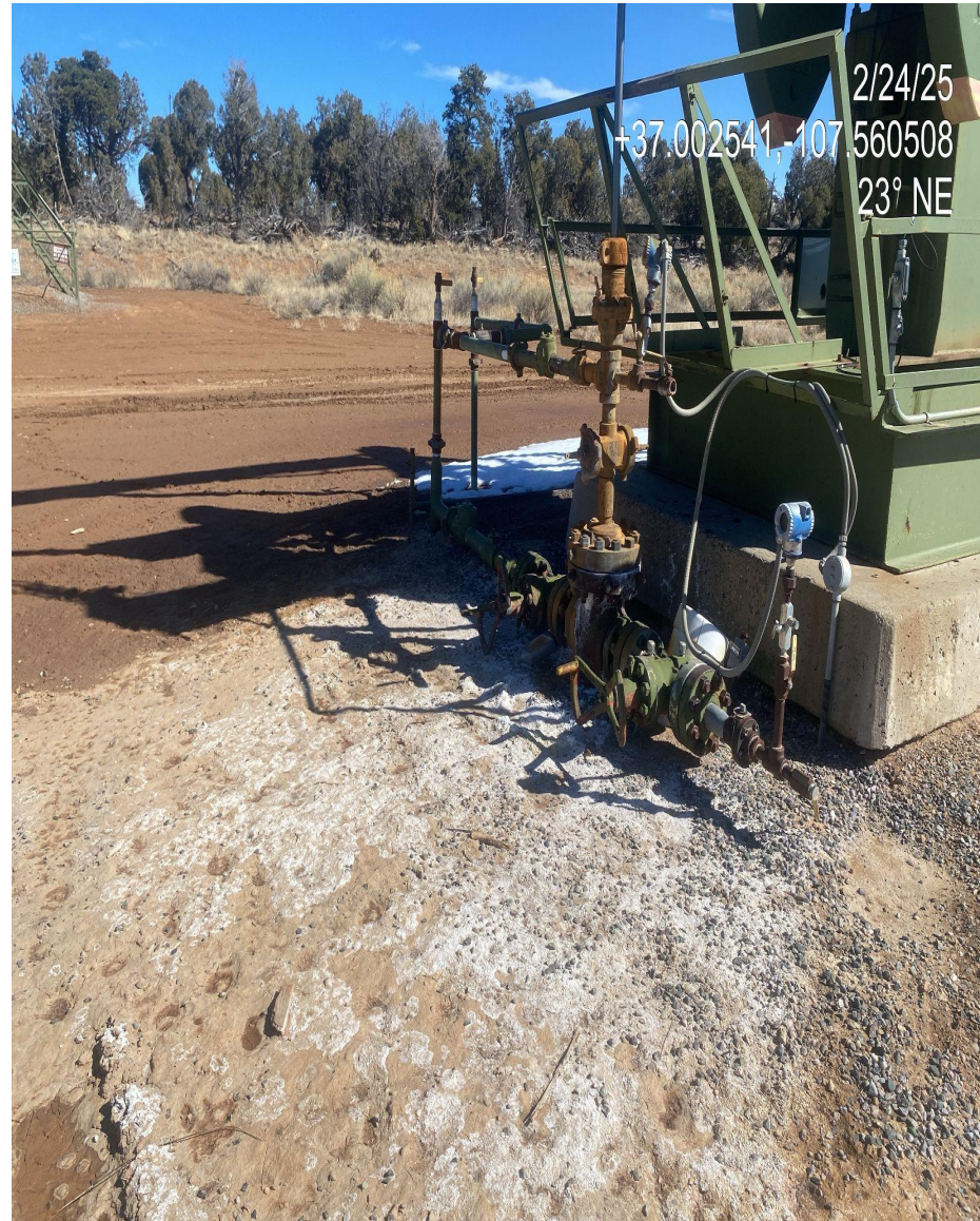
Photo 3. View of salt stain migrating from wellhead.
