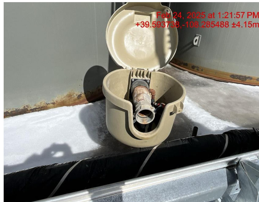
Photo # 5699 Open ended load line
