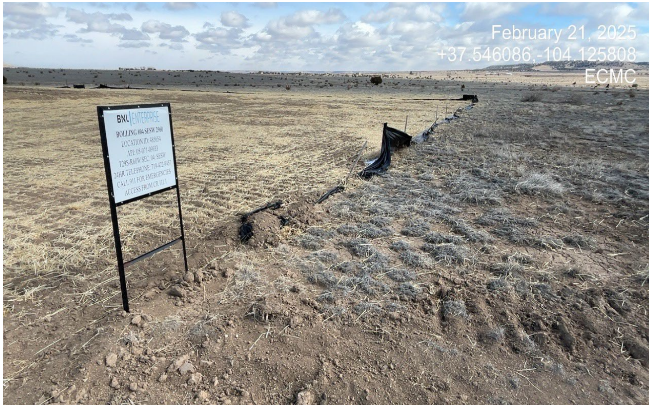
Photo 3. The degraded perimeter silt fence has not been repaired or removed.
