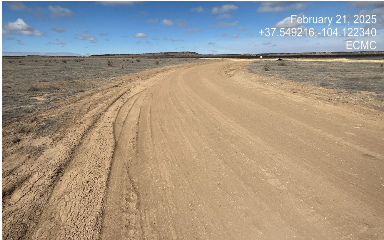
Photo 1. Facing west toward the access road. The side of the road needs to be seeded and stabilized. Previous corrective action was not completed.
