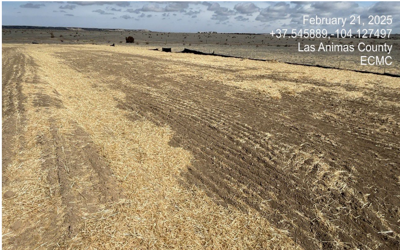
Photo 4. Facing northwest toward the interim reclamation area. Some of the straw mulch has blown off the seeded soil.
