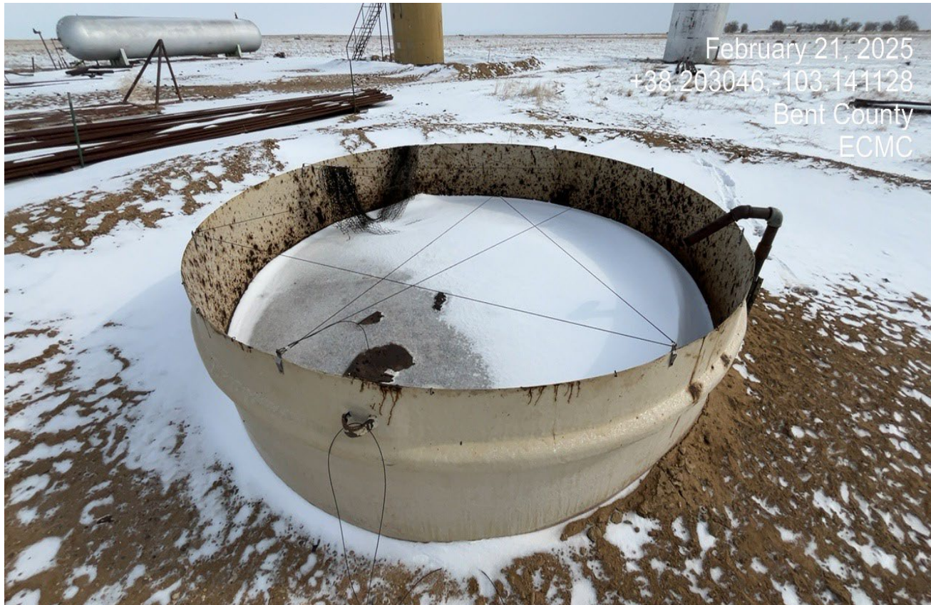
Photo 15. Facing toward the open top tank which has oil condensate inside the tank with no wildlife or livestock protections. The liquids were frozen at the time of inspection. Operator ignored the previous notification and corrective action.
