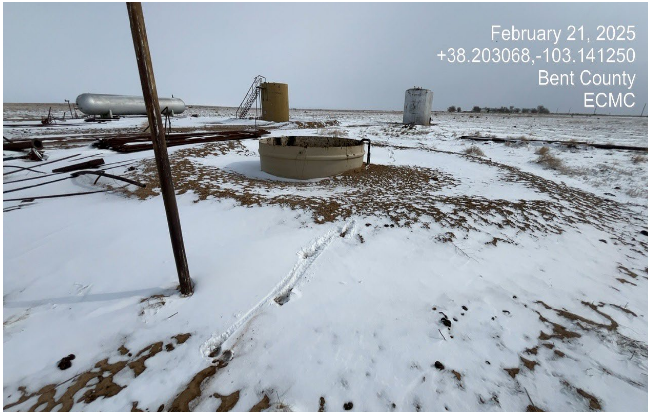
Photo 14. Facing east at the south side of the location. This open top tank remains with oily fluids and a cattle track in the snow goes right up to the tank.
