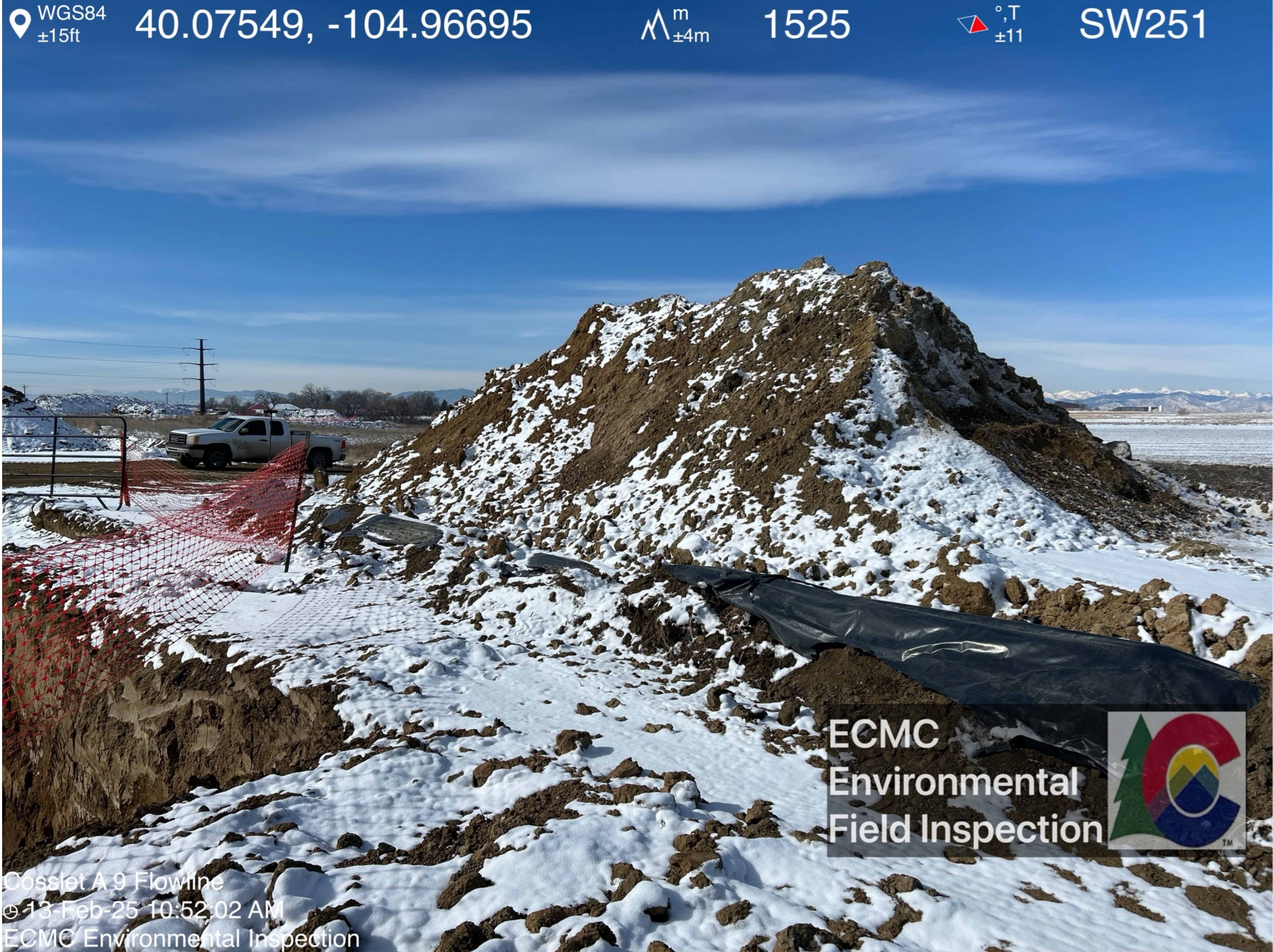
Soil stockpile labeled "contaminated" is on a liner. Snow has covered portions of the stockpile and liner.
