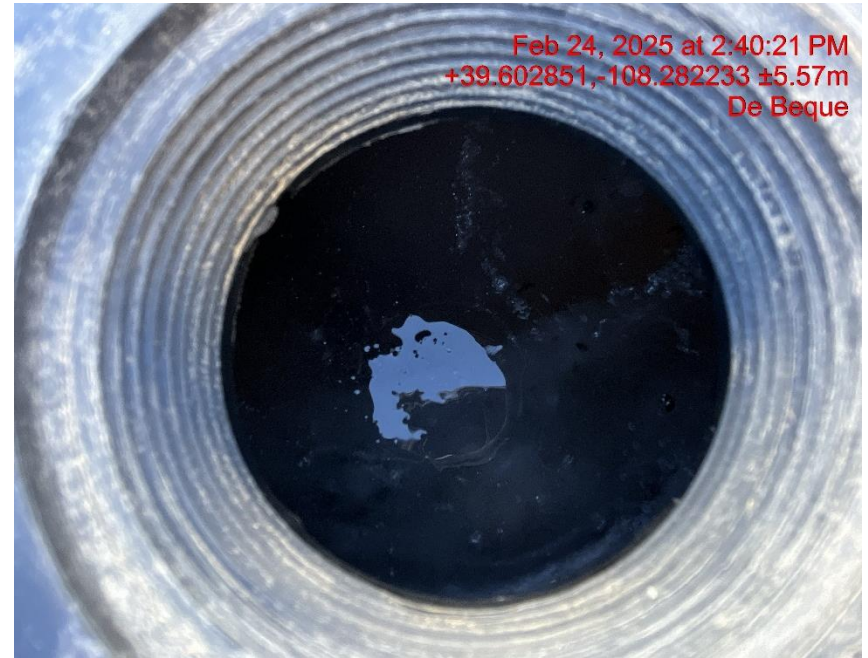
Photo # 5749 Failure to maintain chemical BMP's/chemical containments full of fluid & not sufficient to contain possible spill
