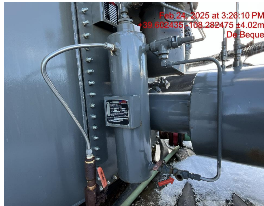
Photo # 5783 PRV vent lines on tank heaters do not comply with CECMC pressure safety device rules
