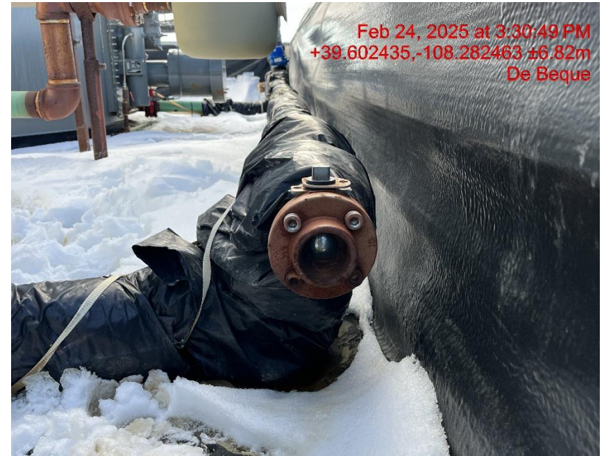
Photo # 5787 Open ended load line
