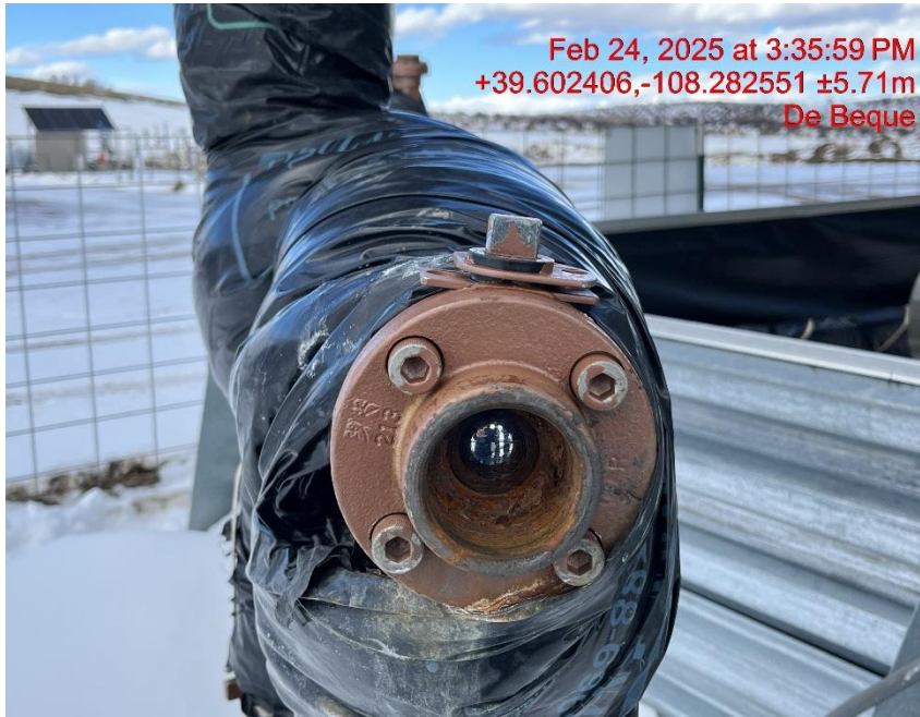
Photo # 5793 Open ended load line
