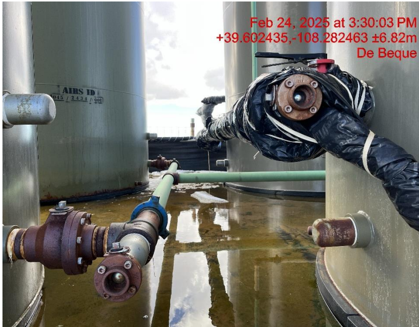
Photo # 5786 Open ended load lines
