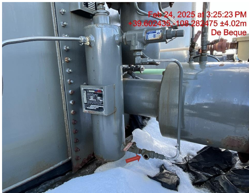
Photo # 5782 PRV vent lines on tank heaters do not comply with CECMC pressure safety device rules
