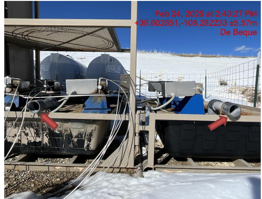
Photo # 5751 Open ended piping on chemical pumps containments/wildlife hazard/available for entry by wildlife
