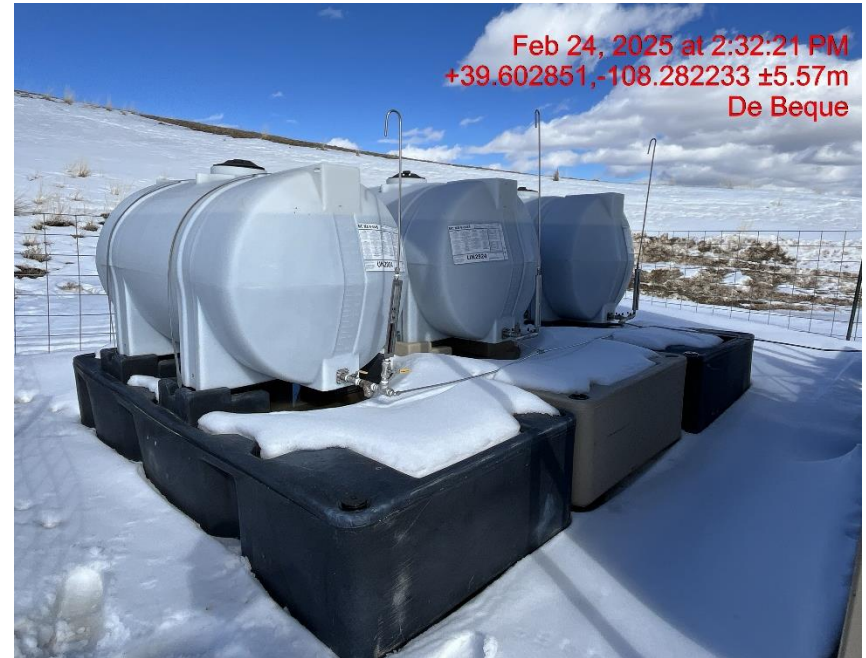
Photo # 5745 Failure to maintain chemical BMP's/chemical containments full of fluid & not sufficient to contain possible spill
