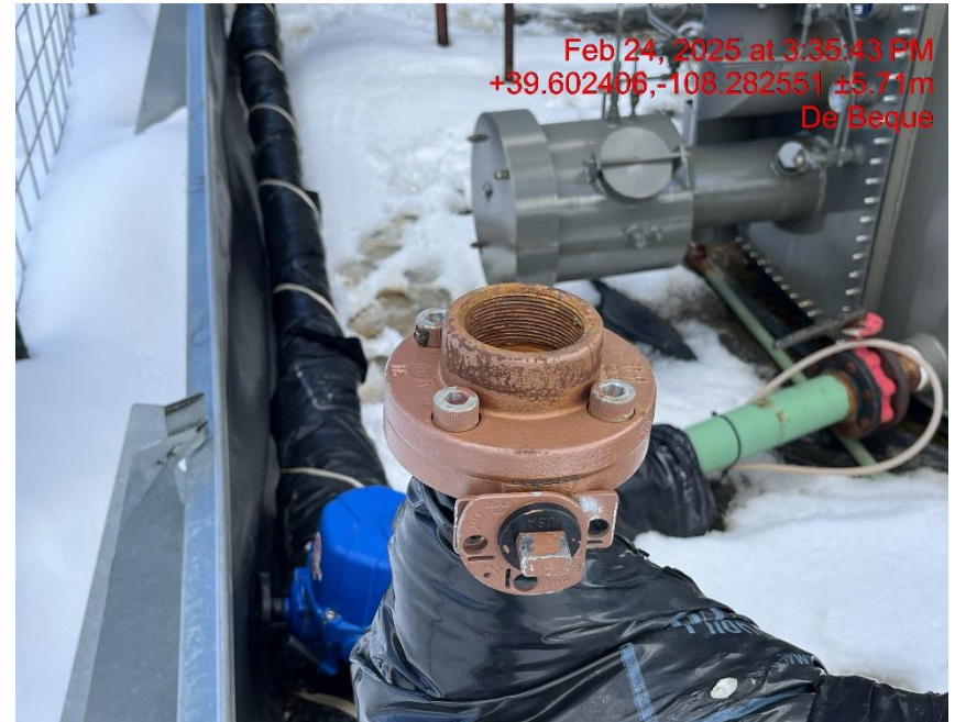
Photo # 5792 Open ended load line
