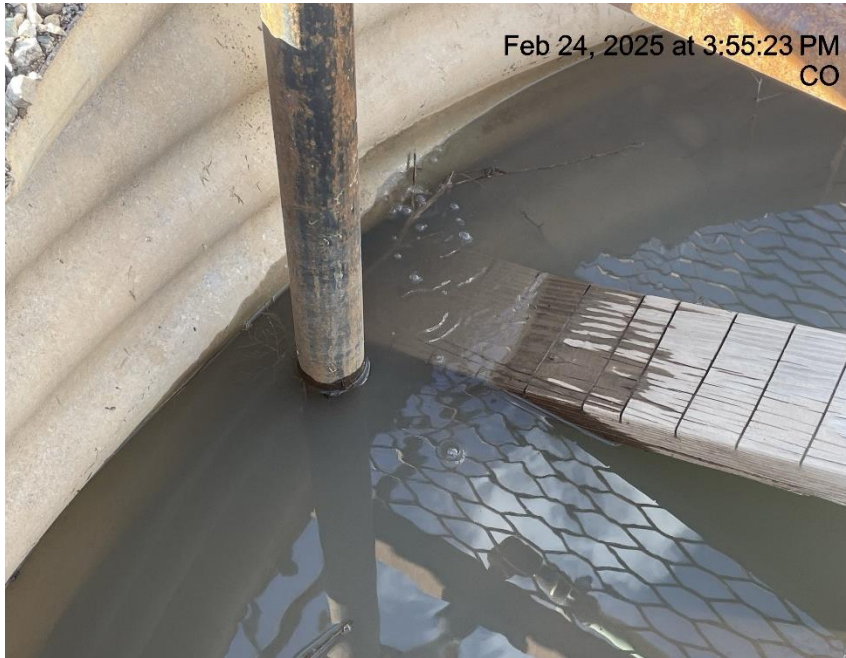
Photo # 8806 Mechanical Condition - Possible leak/gas bubbling up through water in cellar near bradenhead line (HANGS A2 well)
