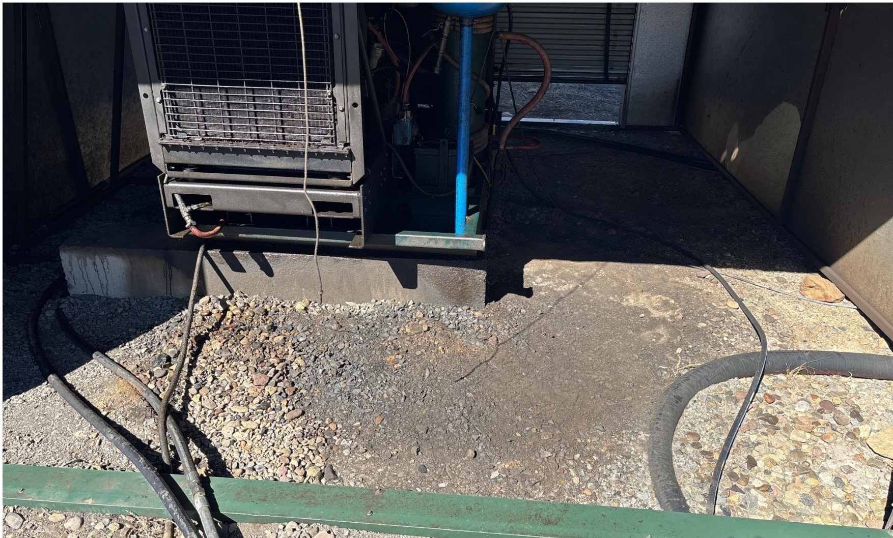
PHOTO 4: LARGE AREA OF IMPACTED SOIL AROUND COMPRESSOR INSIDE AND OUTSIDE OF SOUND MITIGATION SHED. Conduct maintenance on equipment, cleanup stained material and review self inspection processes. COMPLY WITH RULE 1002,(2).D. THIS IS THE SECOND NOTICE FOR THIS CA, IMMEDIATE ACTION IS REQUIRED ( REPAIR LEAKING EQUIPMENT).
