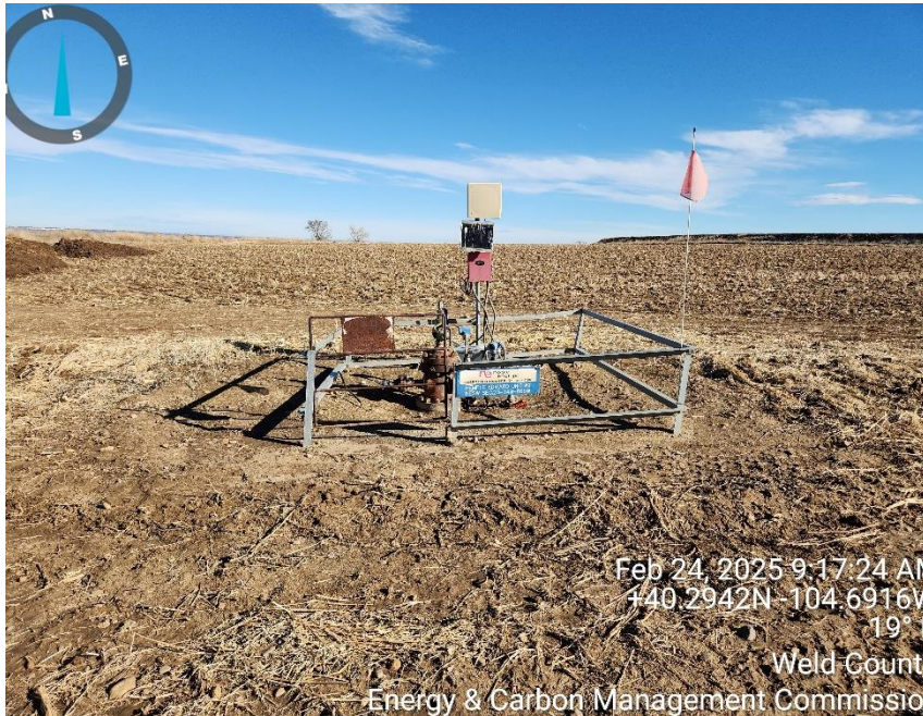
Photo 1 well head and equipment
