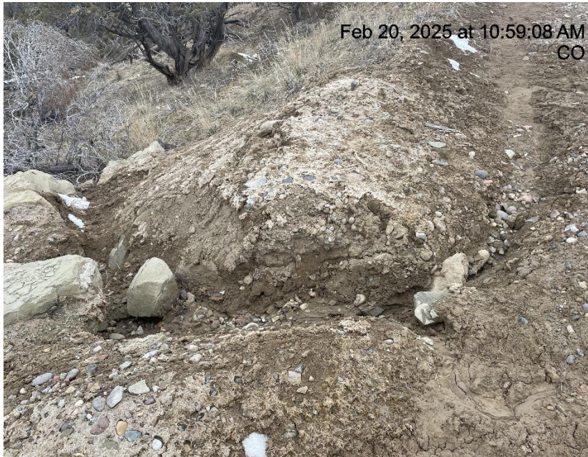
Photo # 7737 Erosion & transport of sediment off location /insufficient BMP's
