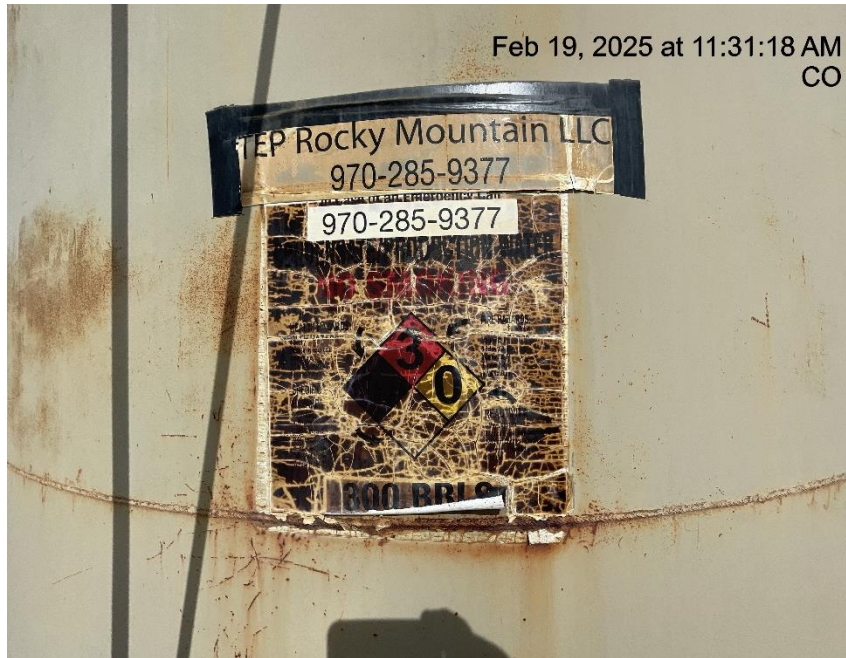
Photo # 6731 Tank label weathered & some required information is illegible
