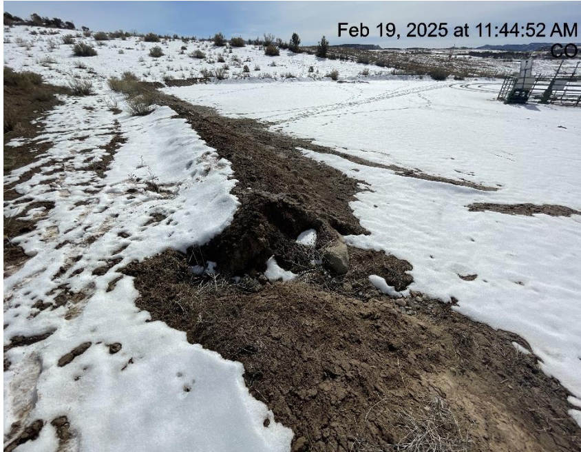
Photo # 6733 Erosion & transport of sediment onto location/berm needs maintenance
