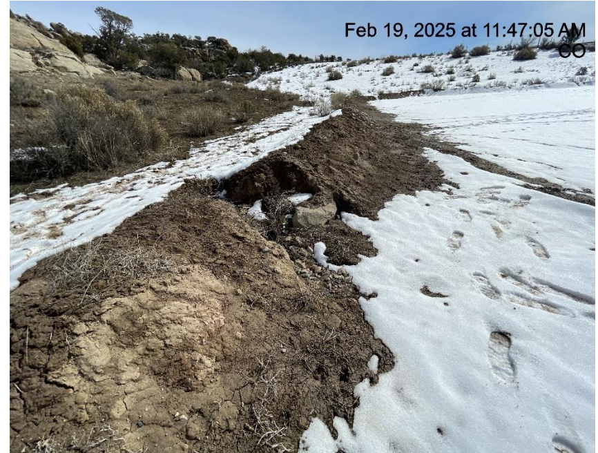
Photo # 6734 Erosion & transport of sediment onto location/berm needs maintenance
