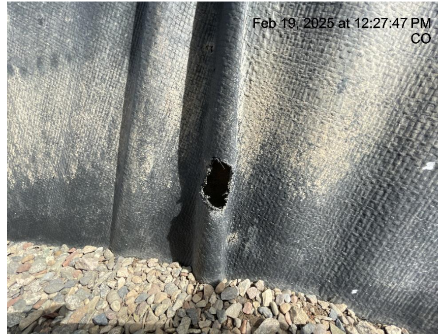
Photo # 6932 Hole in liner/liner needs maintenance
