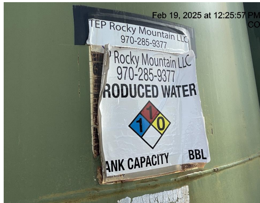
Photo # 6936 Tank label lacks capacity
