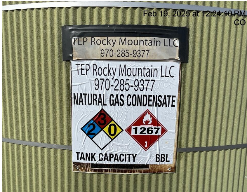
Photo # 6937 Tank label lacks capacity
