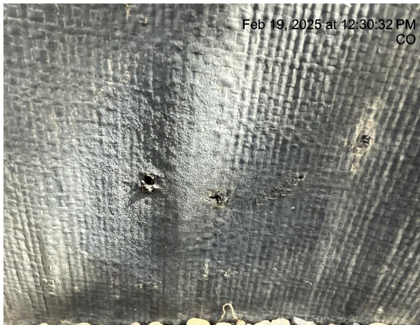
Photo # 6935 Hole in liner/liner needs maintenance
