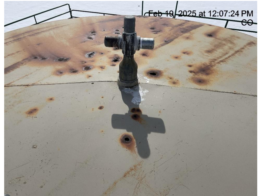
Photo # 6943 Multiple holes in tank/tank lacks integrity
