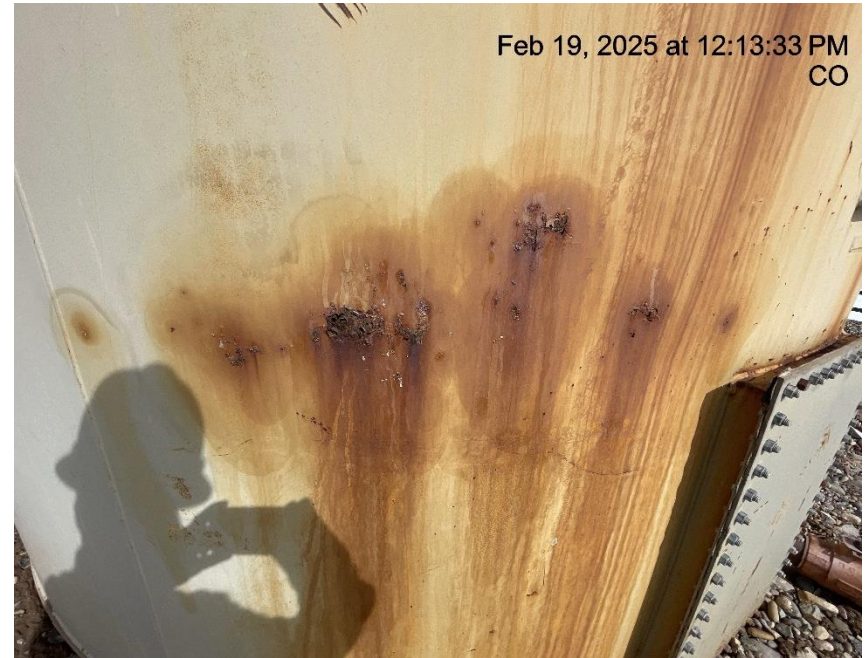
Photo # 6941 Multiple holes in tank/tank lacks integrity
