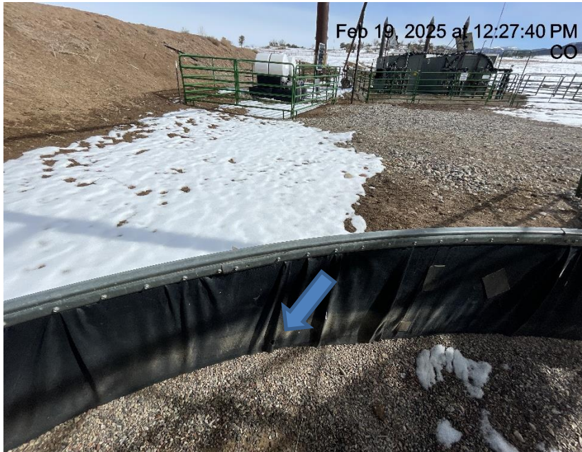
Photo # 6931 Hole in liner/liner needs maintenance
