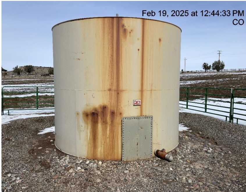
Photo # 6940 Multiple holes in tank/tank lacks integrity
