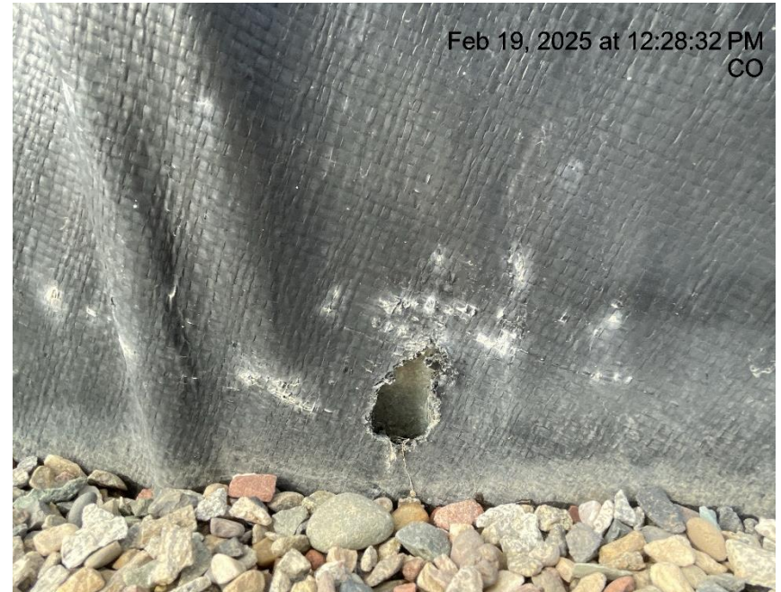
Photo # 6934 Hole in liner/liner needs maintenance
