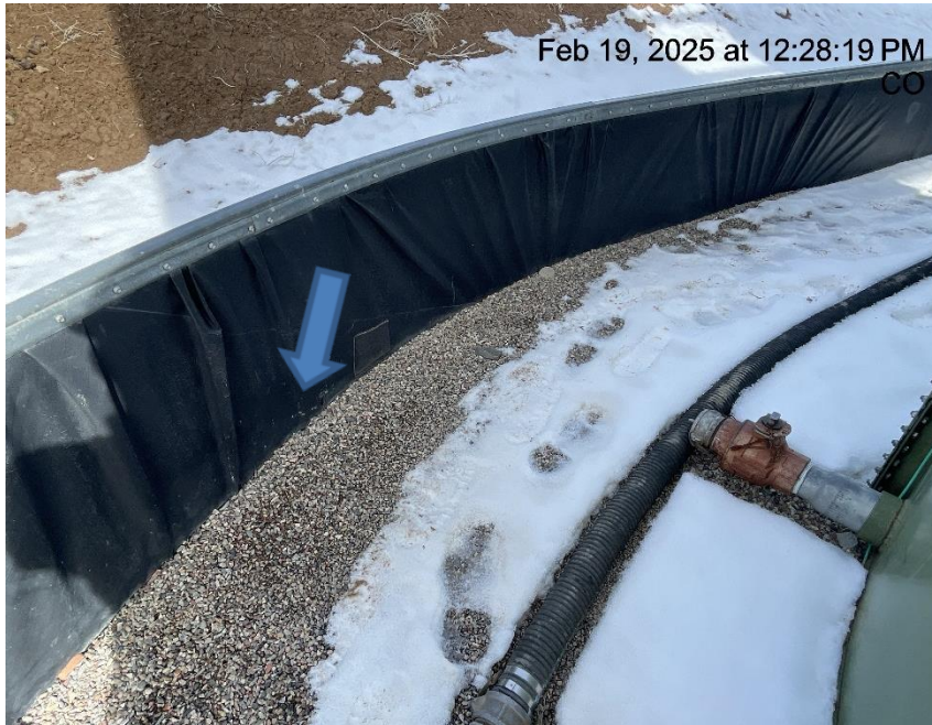
Photo # 6933 Hole in liner/liner needs maintenance
