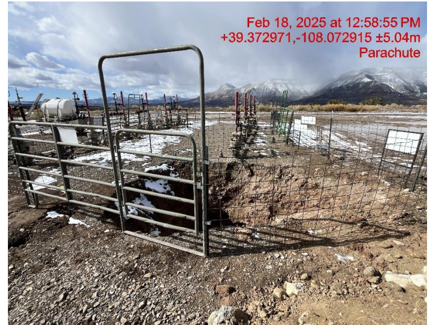
Photo # 5223 Open hole with no wildlife egress/wildlife hazard
