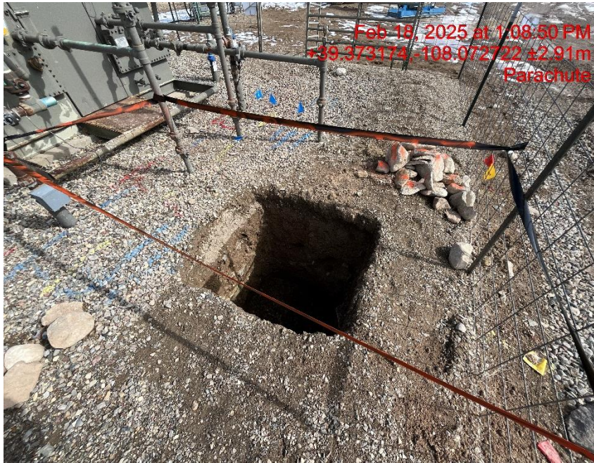
Photo # 5236 Open hole with no wildlife egress/wildlife hazard
