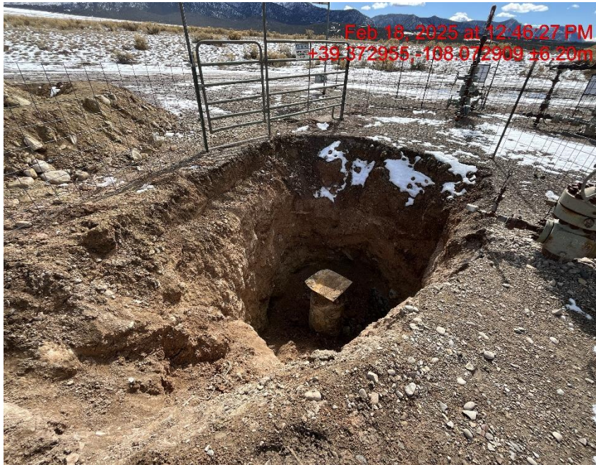
Photo # 5213 Open hole with no wildlife egress/wildlife hazard
