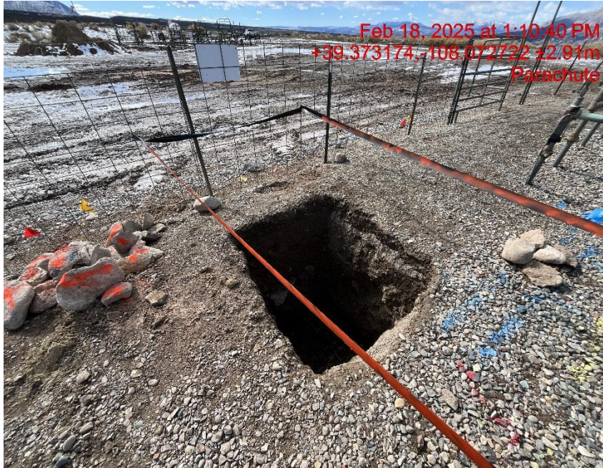
Photo # 5238 Open hole with no wildlife egress/wildlife hazard
