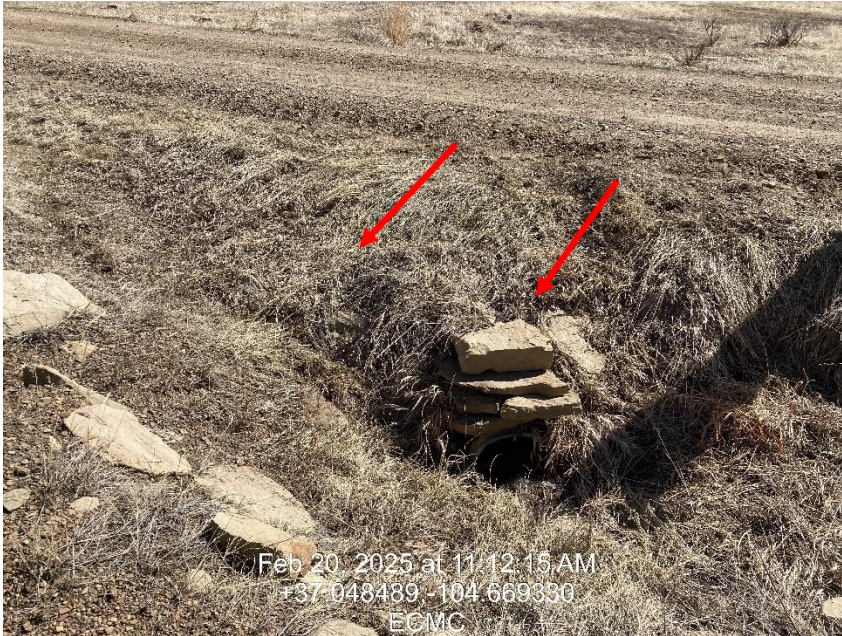
Photo 13 – Culvert in road, direction change
