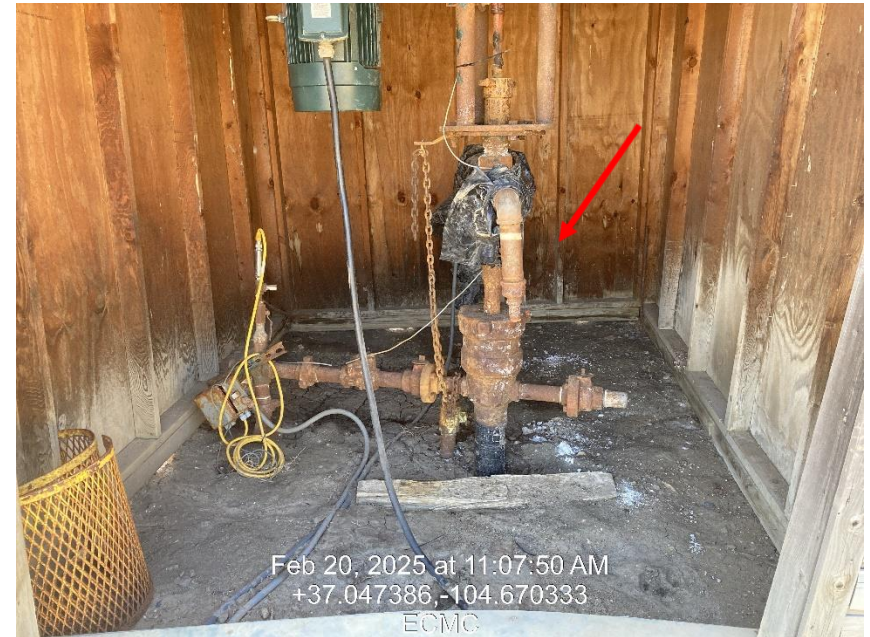
Photo 4 – Wellhead, white stained soils are present.
